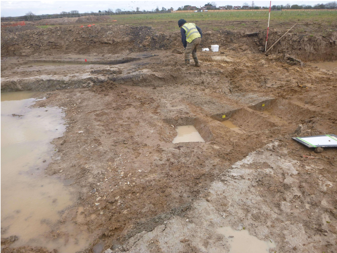
Photograph 8 Drainage ditches F186, F188 and F189 in Area 2 after L7 had been removed – view north-east.
