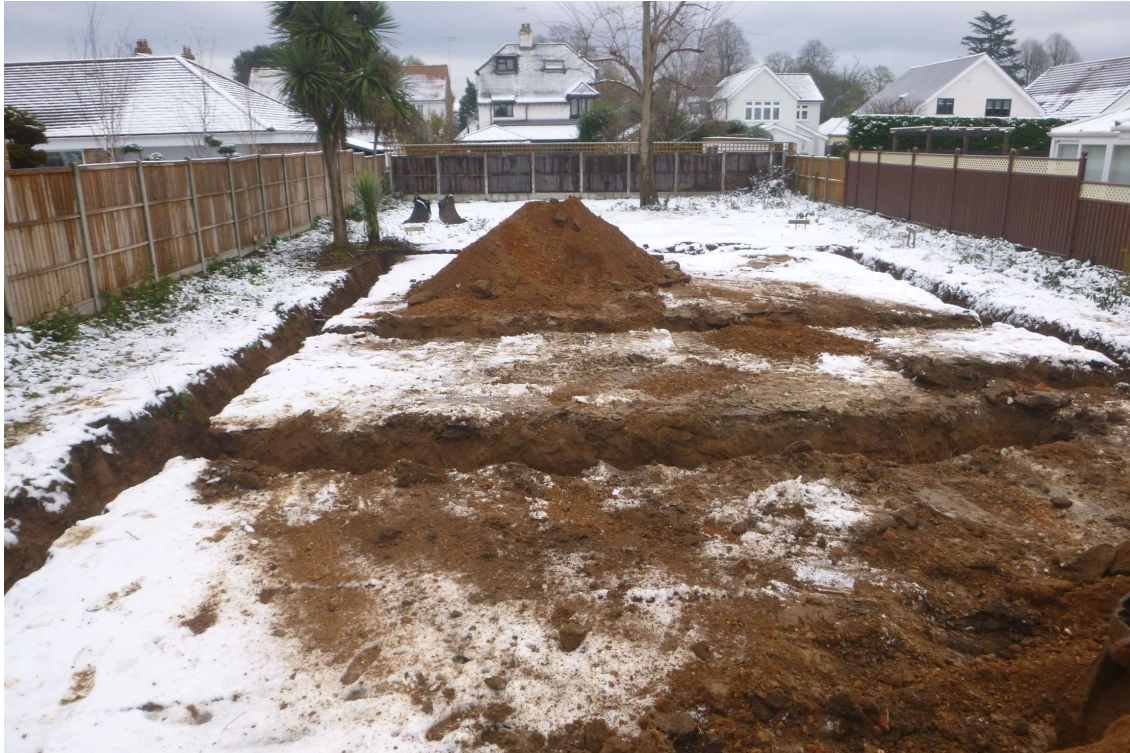
Photograph 1 Bungalow foundation trenches, looking east.
