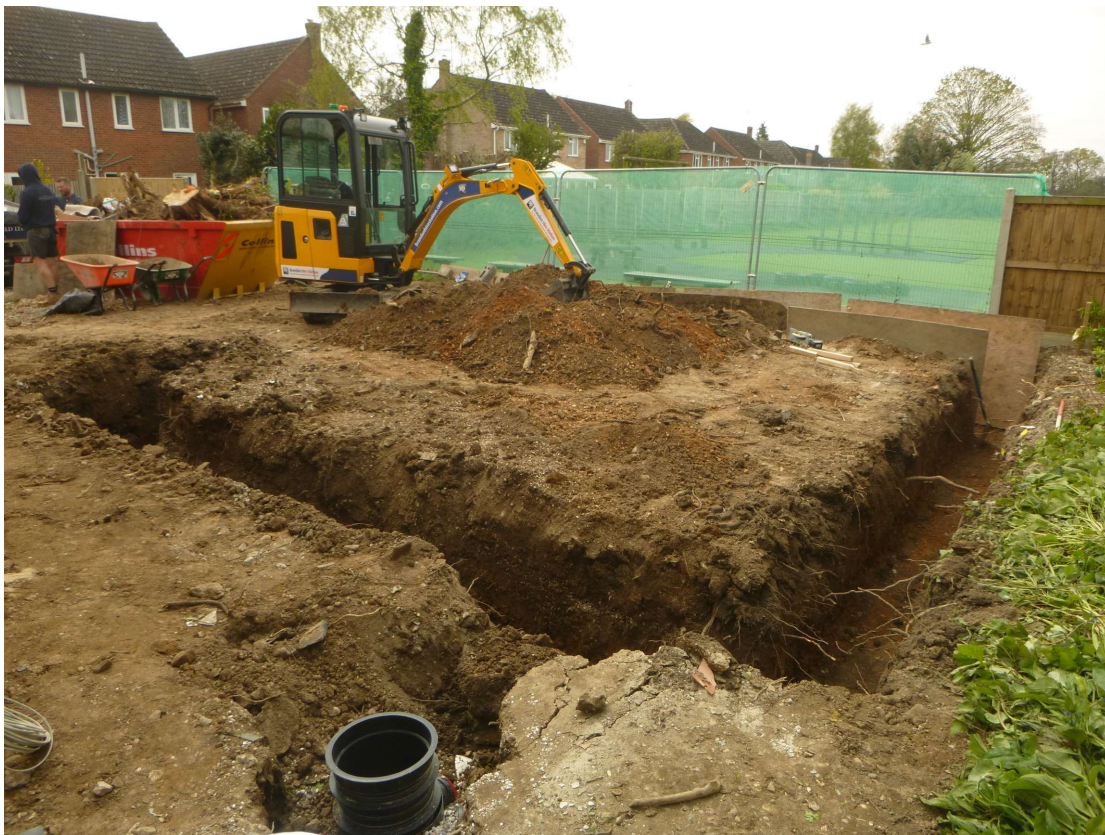
Photograph 4 Garage foundation trench, looking south-west.
