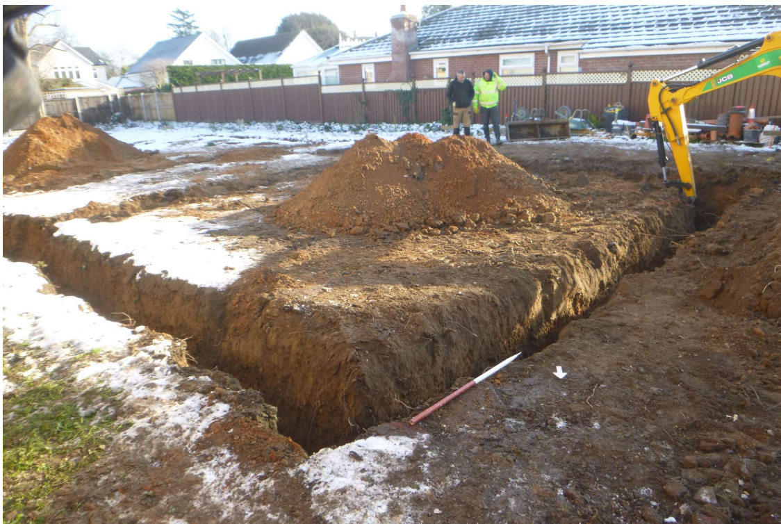
Photograph 2 Bungalow foundation trenches, looking south-east.
