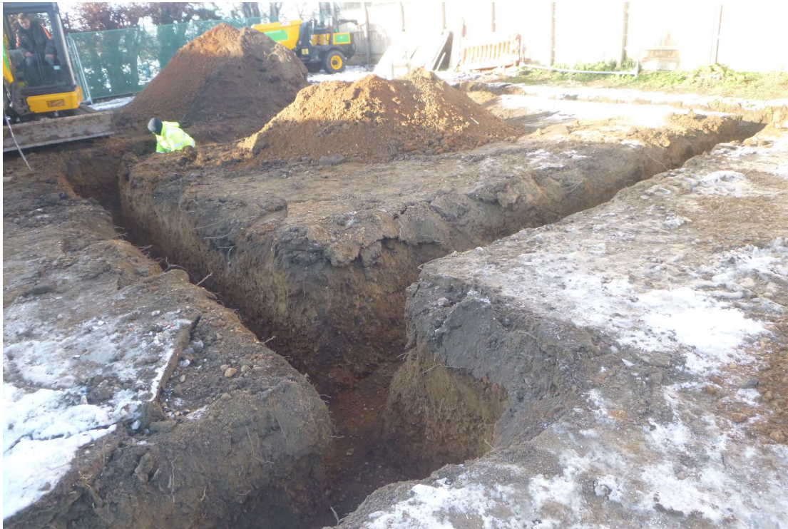
Photograph 3 Bungalow foundation trenches, looking north-west.
