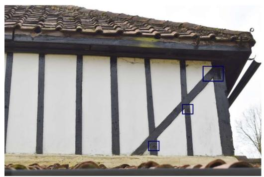
Photograph 4 Detail of carpenters' marks (outlined in blue) on northern elevation of barn (upper register). 'IIII' on the principal post and the two studs to the left. Also, detail of reused timber for corner post. Photograph taken facing south.
