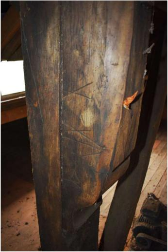
Photograph 28 Detail of Baltic timber marks on post between bays 6 and 7 of barn.
