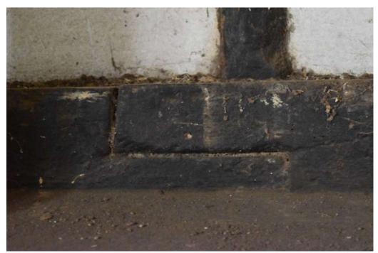
**Photograph 21** Detail of side-halved scarf joint in northern sill-beam in bay 1 of barn. Photograph taken facing north-west.
