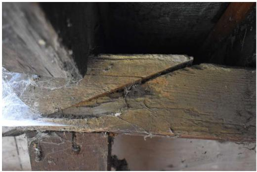
**Photograph17** Detail of splayed scarf joint in purlin on eastern roof pitch of barn, between bays 6 and 7. Photograph taken facing north-east.
