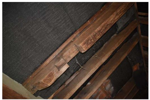
**Photograph 15** Example of notch in rafter from removed purlin and Baltic timber mark in western roof pitch of barn (between bays 5 and 6). Photograph taken facing north-west.
