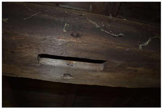
**Photograph 16** Example of empty mortice from removed brace in tie-beam (between bays 6 and 7) of barn. Photograph taken facing east south-east.
