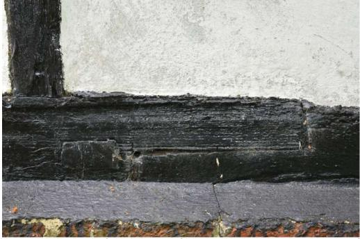
**Photograph 14** Detail of side-halved scarf joint in sill-beam on southern elevation of barn. Photograph taken facing north north-west.
