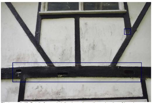
**Photograph 13** Detail of reused girding-beam in southern elevation of barn (upper register). carpenters' mark 'II' on right-hand stud. Both outlined in blue. Photograph taken facing north north-west.
