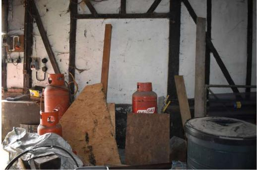
**Photograph 23** Detail of inserted and blocked opening in bay 5 of barn, ground floor. Photograph taken facing north-east.
