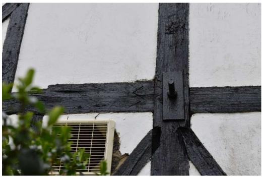
Photograph 11 Detail of carpenters' marks 'VI' on girding-beam on western elevation of barn. Photograph taken facing east north-east.
