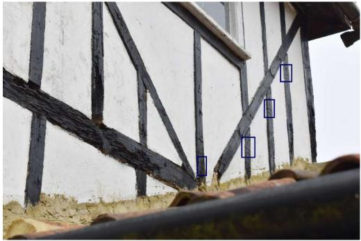
Photograph 3 Detail of carpenters' marks on eastern elevation of barn (upper register). XX on the central stud and 'XII' on last three studs (outlined in blue). Photograph taken facing west.
