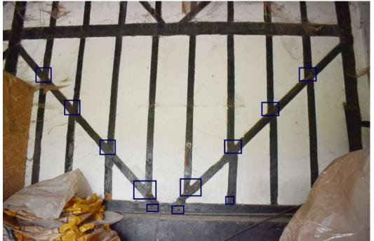
**Photograph 5** Detail of northern elevation of barn (lower register) visible in stable 4. carpenters' marks outlined in blue. Photograph taken facing southeast.
