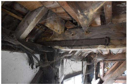
**Photograph 18** Example of tie-beam iron strap (eastern end of tie-beam between bays 1 and 2). Photograph taken facing east.
