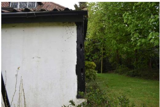
Photograph 10 Detail of reused corner post on western elevation of barn extension. Photograph taken facing north-east.
