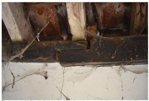
**Photograph 26** Detail of side-halved scarf joint in western wall-plate of bay 3 of barn. Photograph taken facing north-east.
