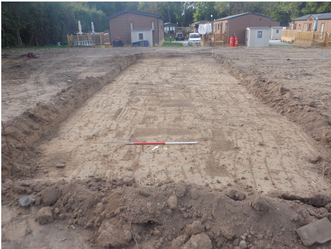
Photograph 3 Foundation pad 2, looking north-west.
