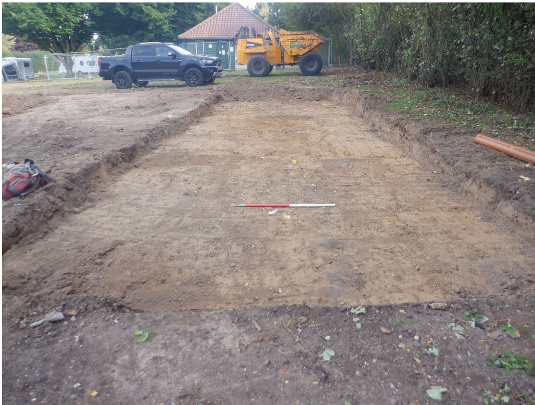
Photograph 1 Foundation pad 1, looking south-east.
