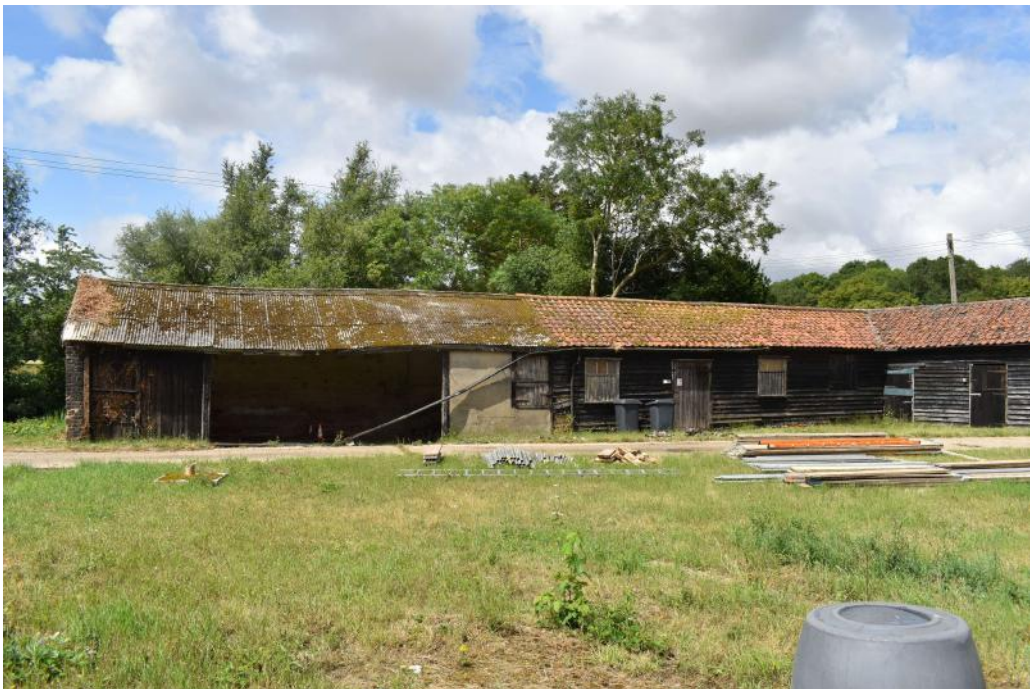
Photograph 29 North-east elevation of Pond Barn. Photograph taken facing south-west.
