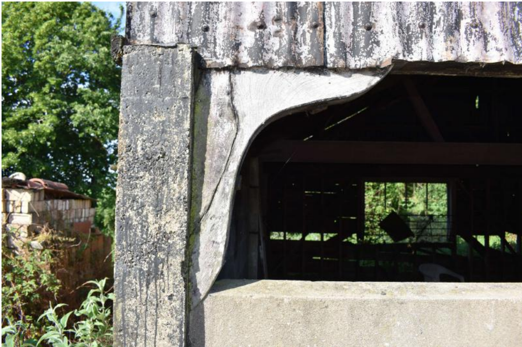
Photograph 40 Detail of knee-brace on north-east elevation of Field Barn. Photograph taken facing south-west.
