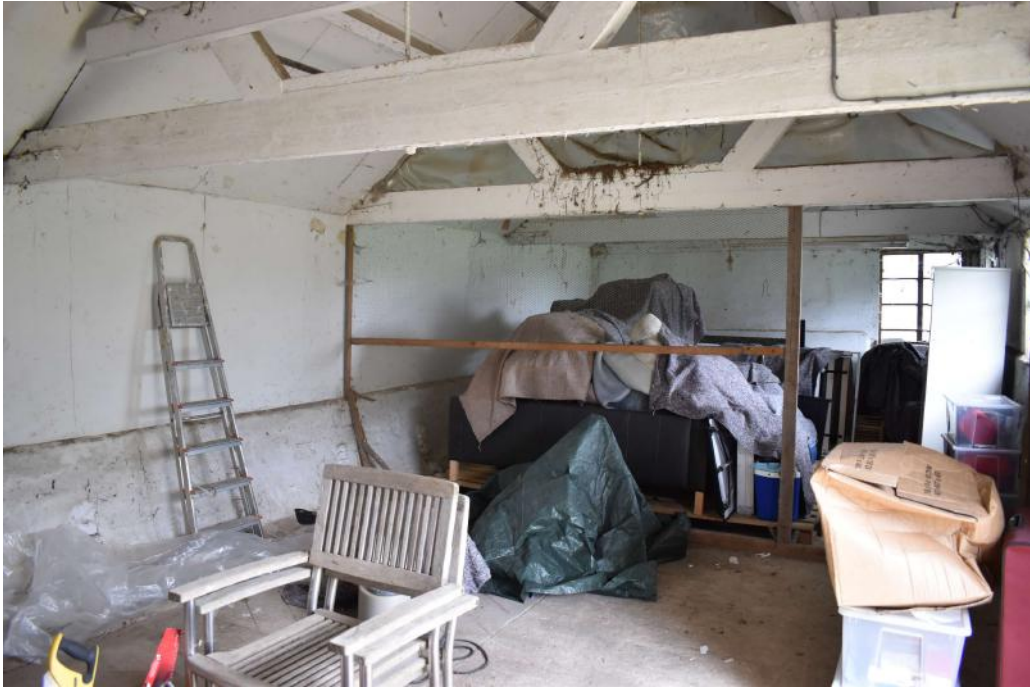
Photograph 17 Interior of Bailey Barn (building 1). Photograph taken facing north.
