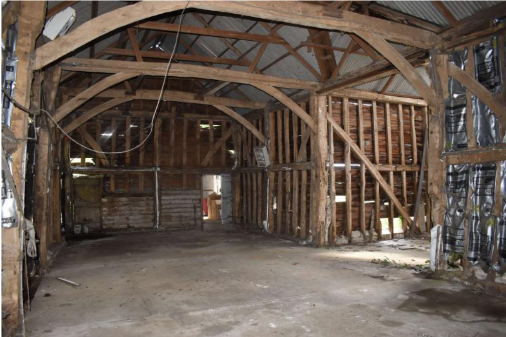
Photograph 6 Interior of Bailey Barn (threshing barn). Photograph taken facing north-east.
