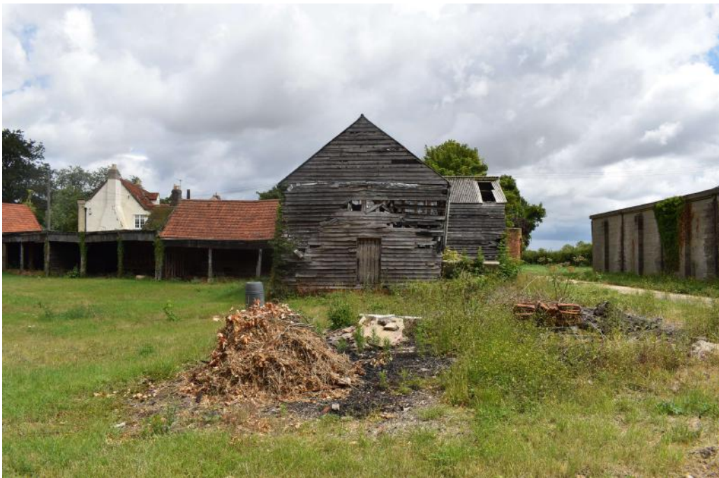
Photograph 5 South-west elevation of Bailey Barn. Photograph taken facing north-east.
