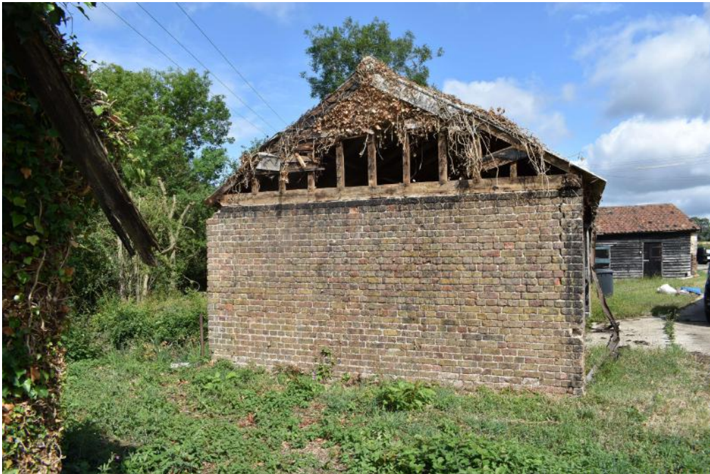
Photograph 30 South-east elevation of Pond Barn. Photograph taken facing north-west.
