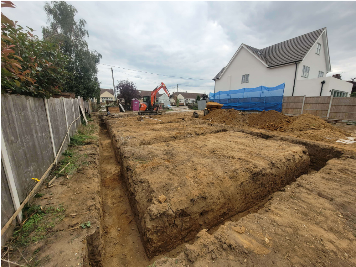
Photograph 2 Foundation trenches, looking south-east.
