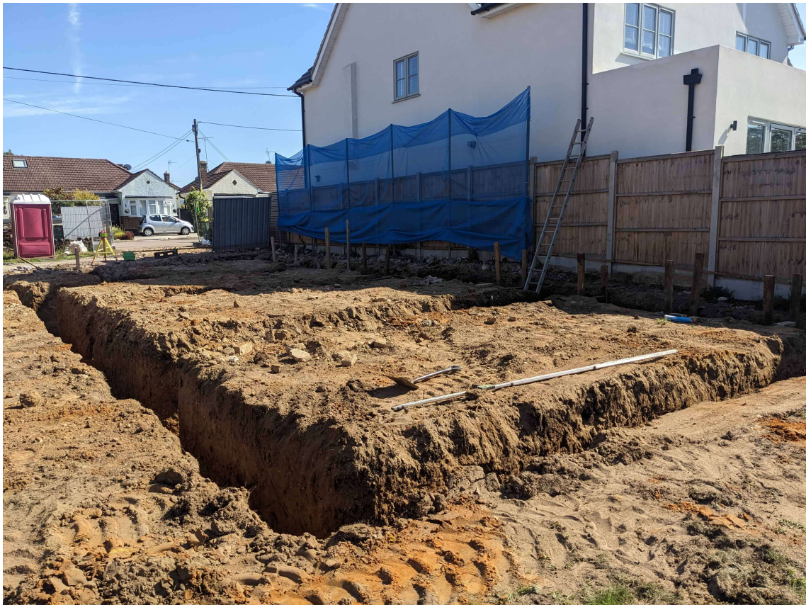
Photograph 1 Foundation trenches, looking south-east.
