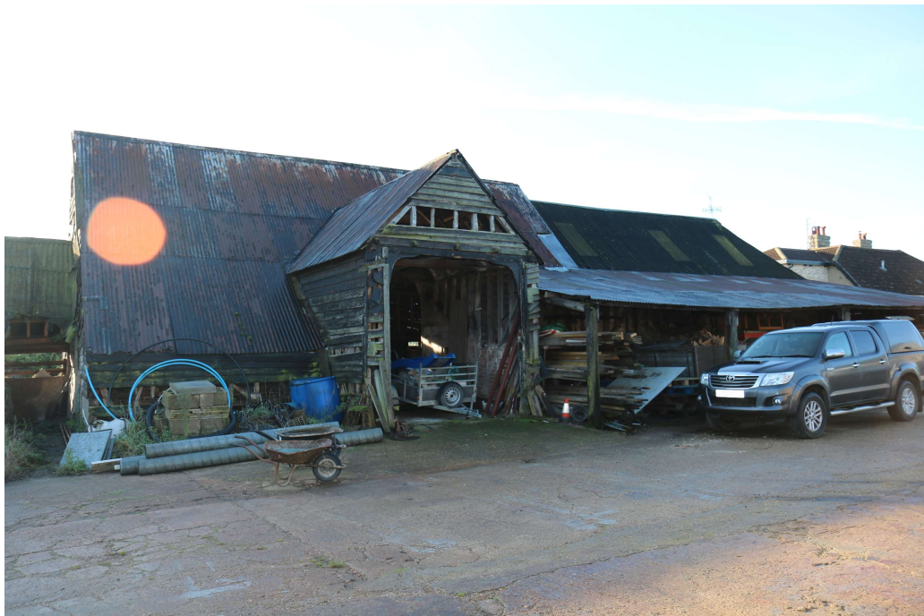
Photograph 1 Northern elevation. Photograph taken facing south south-west.
