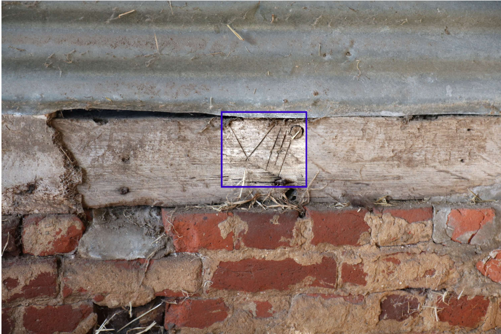
Photograph 28 Detail of carpenter's mark on western sill-beam of bay 2 of four-bay building A. Photograph taken facing south-west.
