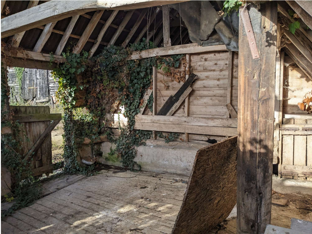
Photograph 33 Interior of six-bay building (bays 5-6). Photograph taken facing north-west.
