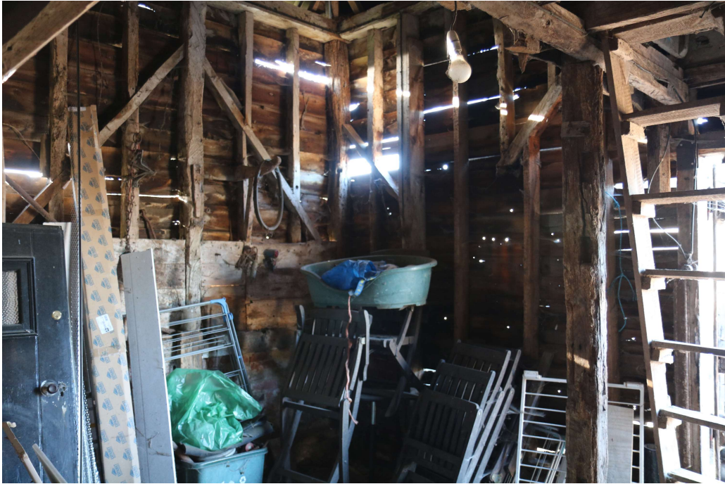
Photograph 22 Interior of four-bay building A (bay 1). Photograph taken facing south-west.
