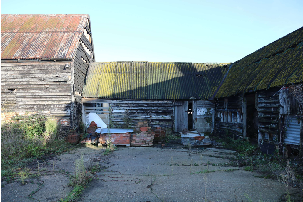
Photograph 6 Southern elevation of four-bay building B. Photograph taken facing west north-west.
