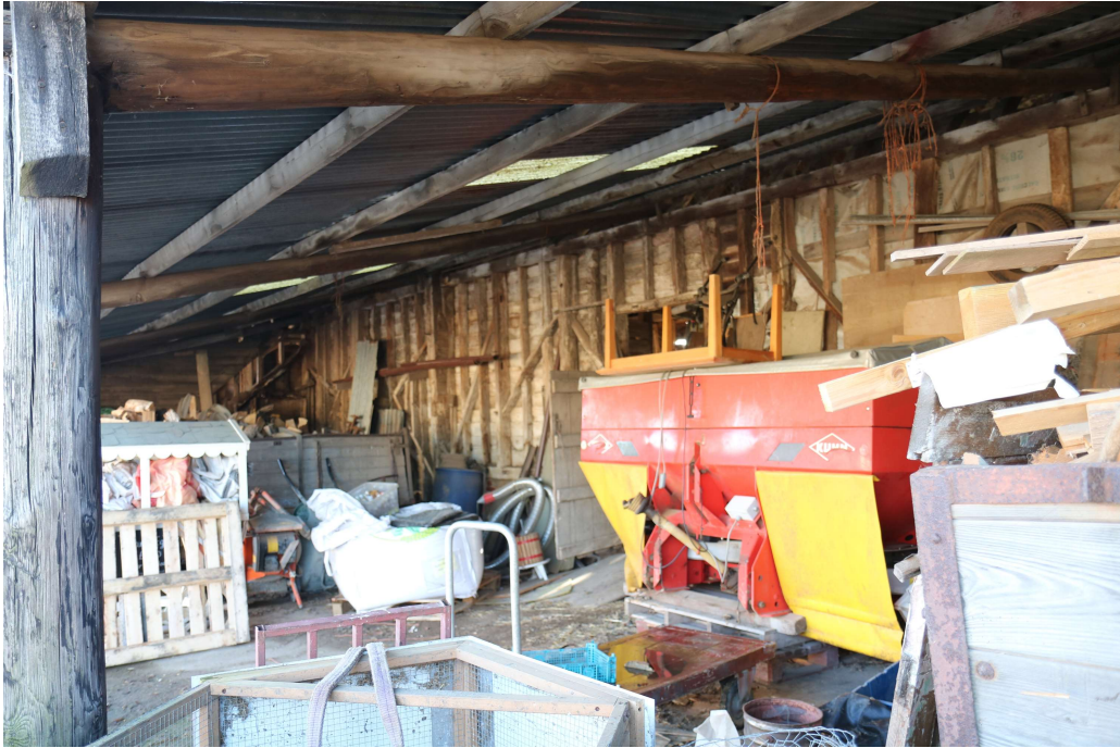
Photograph 34 Interior of lean-to 1. Photograph taken facing south-east.
