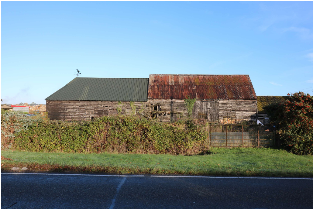
Photograph 4 Southern elevation. Photograph taken facing west north-west.
