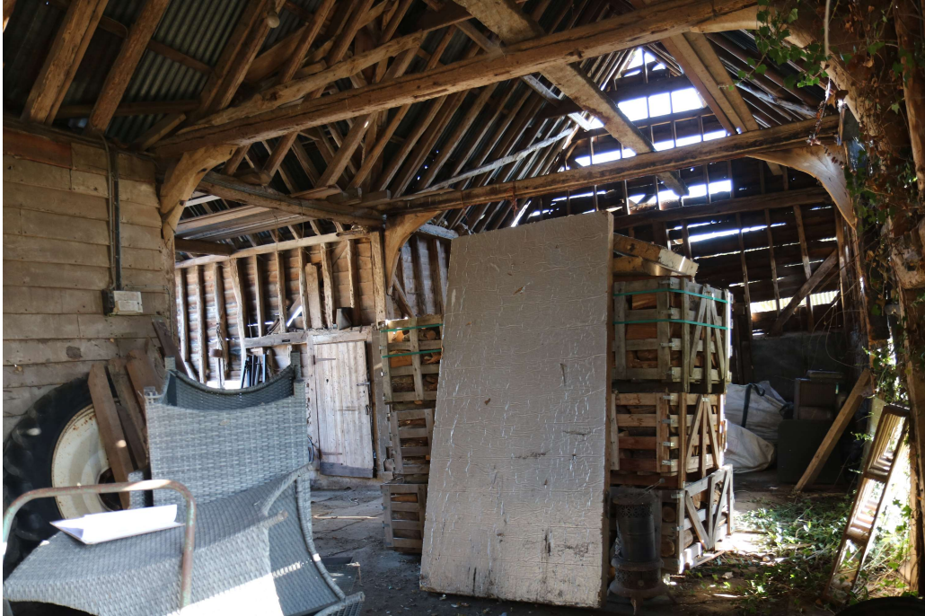
Photograph 10 Interior of threshing barn. Photograph taken facing north-east.
