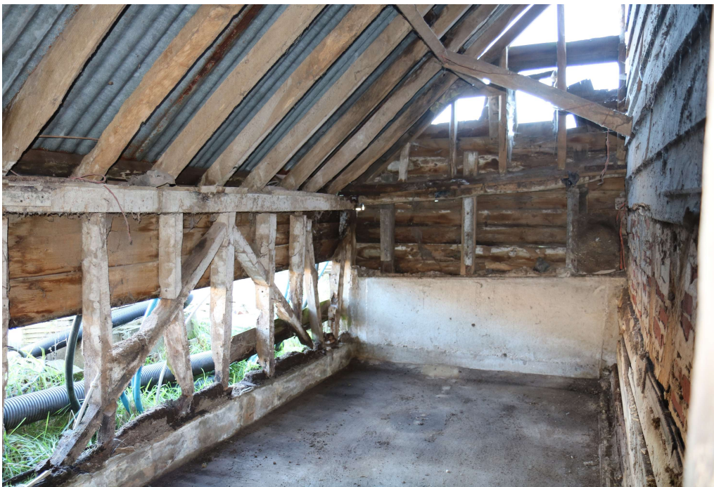
Photograph 35 Interior of lean-to 2. Photograph taken facing north-east.
