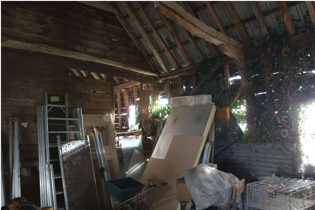
Photograph 29 Interior of four-bay building A (bays 2-4). Photograph taken facing east south-east.
