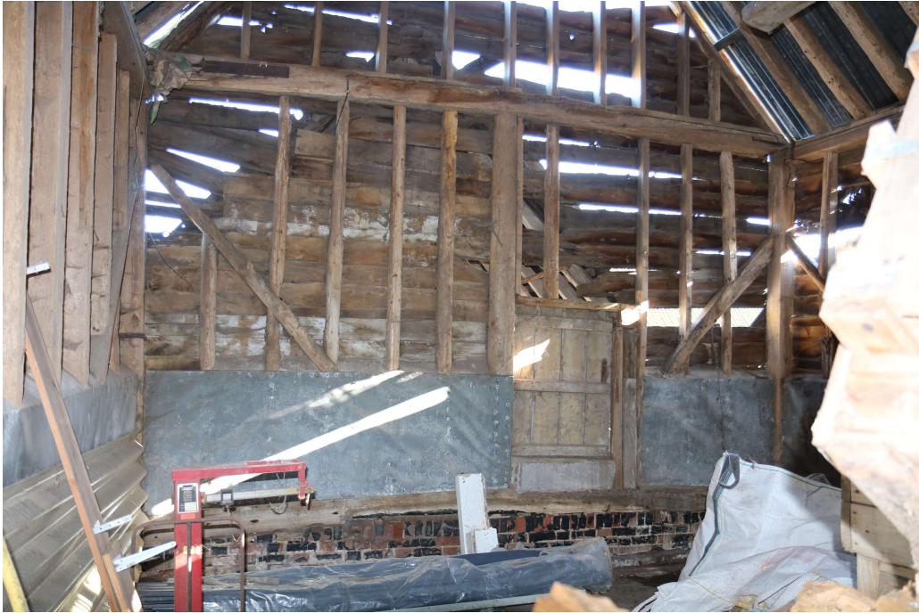
Photograph 17 Eastern wall of bay 3 of threshing barn. Photograph taken facing east.
