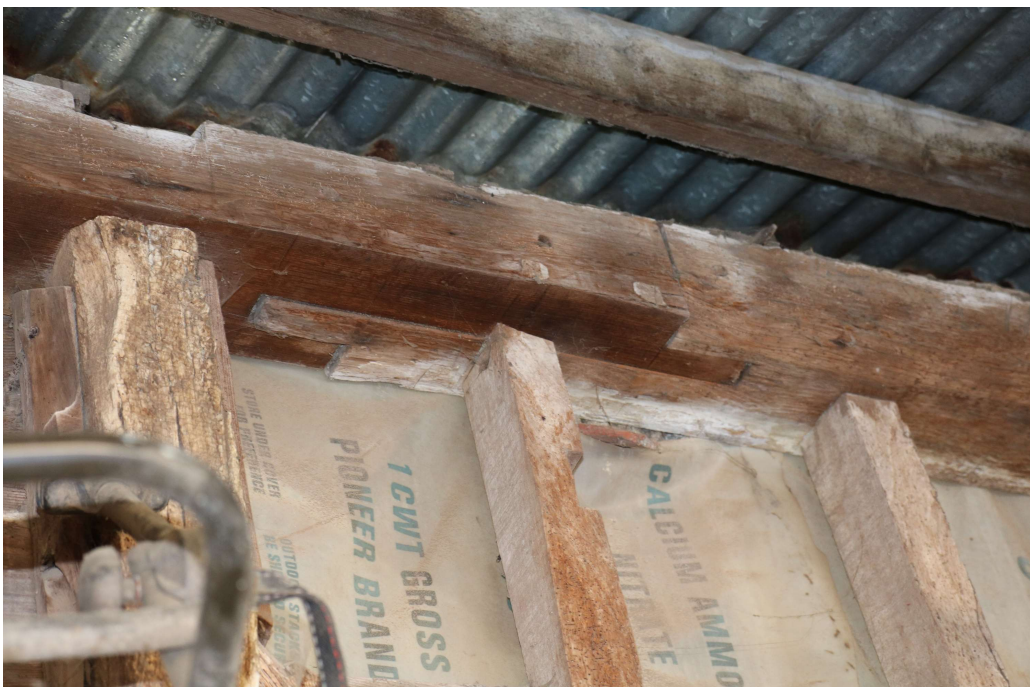
Photograph 27 Detail of scarf joint in northern wall-plate in four-bay building A. Photograph taken facing south-east.
