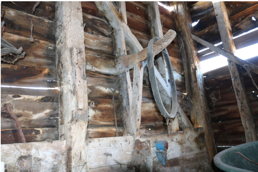
Photograph 23 Detail of saddle hook in four-bay building A (bay 1). Photograph taken facing south-east.
