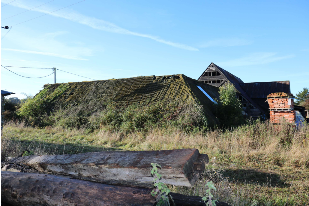
Photograph 3 Eastern elevation. Photograph taken facing south-west.
