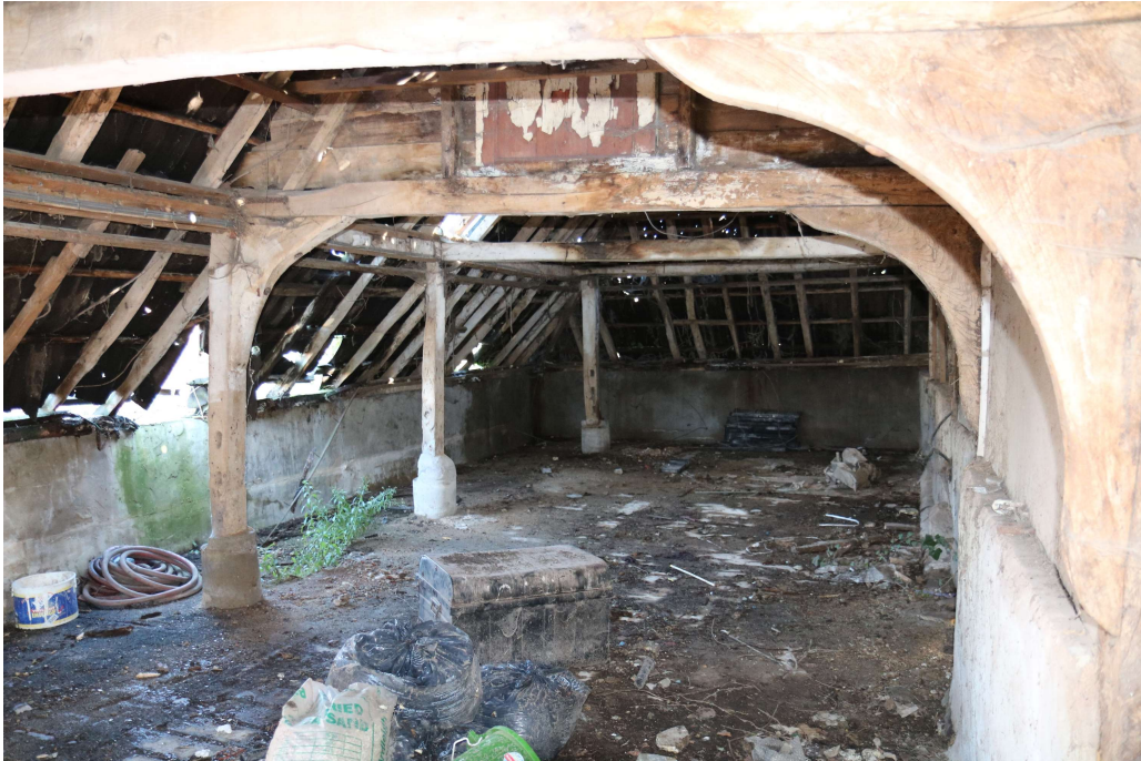
Photograph 30 Interior of four-bay building B. Photograph taken facing north-east.
