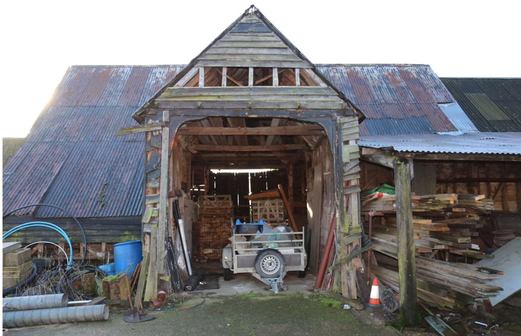
Photograph 2 Northern elevation. Photograph taken facing south south-east.
