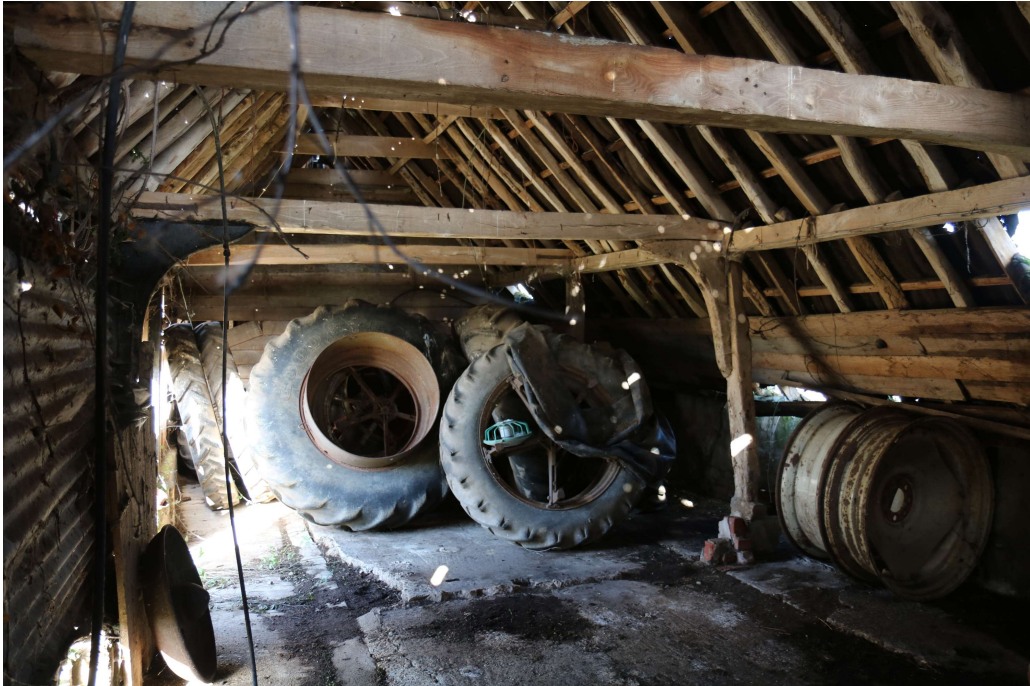
Photograph 31 Interior of six-bay building (bays 1-4). Photograph taken facing north-east.
