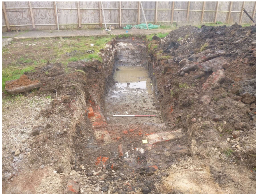
Photograph 3 T5 trench shot – looking south south-west.
