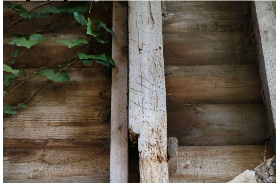
SSGH24 Photograph_056Detail of pintle on post in south-west wall of barn. Photograph take...
