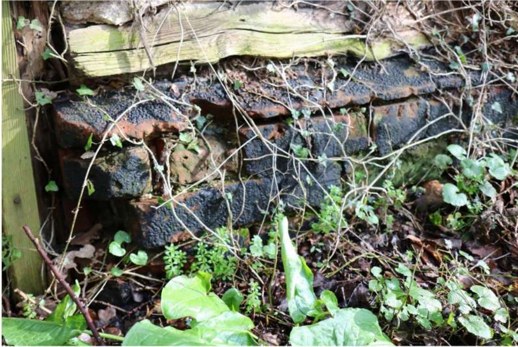
Photograph 2 Detail of brick plinth on south-west elevation. Photograph taken facing east.
