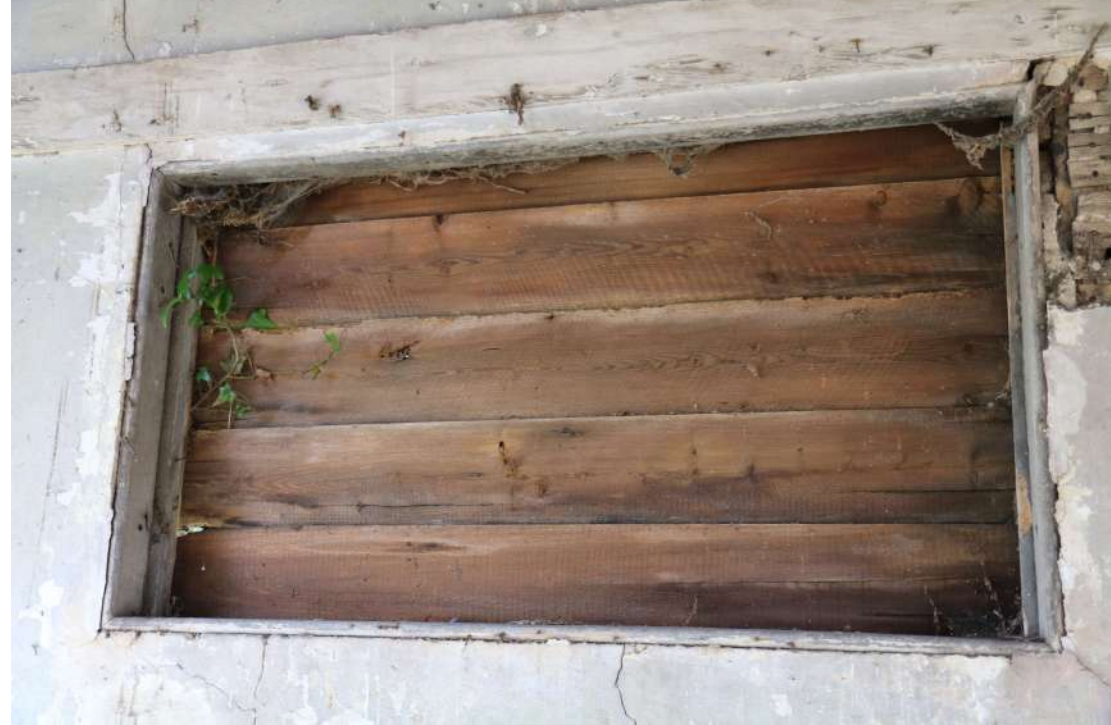
SSGH24 Photograph_031Detail of blocked window in south-east wall of store. Photograph ta...
