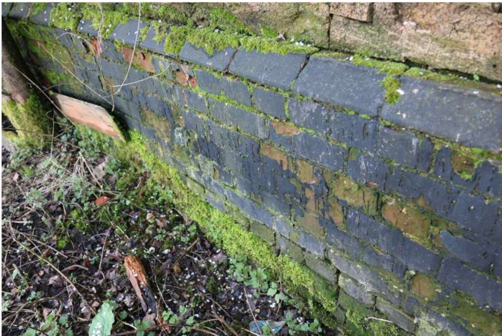
Photograph 3 Detail of brick plinth on north-east elevation. Photograph taken facing south.
