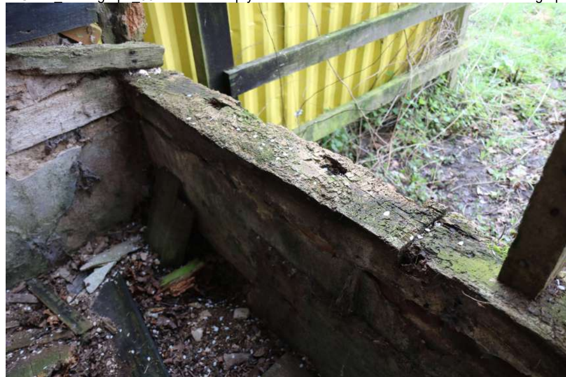
SSGH24 Photograph_052Detail of empty mortices in north-east sill-beam of barn. Photograp...
