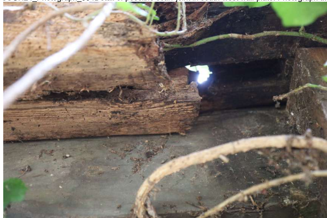
SSGH24_Photograph_036Detail of empty mortice in centre of south-western doorway. Photo...
