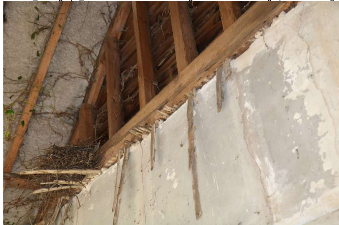
SSGH24 Photograph 039Detail of remains of ceiling laths in store. Photograph taken facing ...
