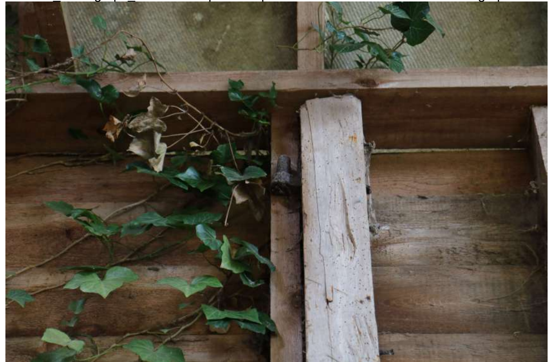
SSGH24 Photograph_056Detail of pintle on post in south-west wall of barn. Photograph take...
