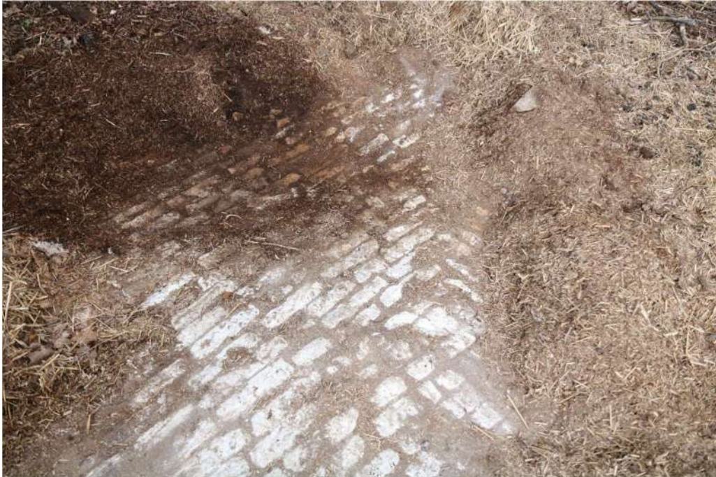
Photograph 10 Detail of brick floor of barn. Photograph taken facing south.
