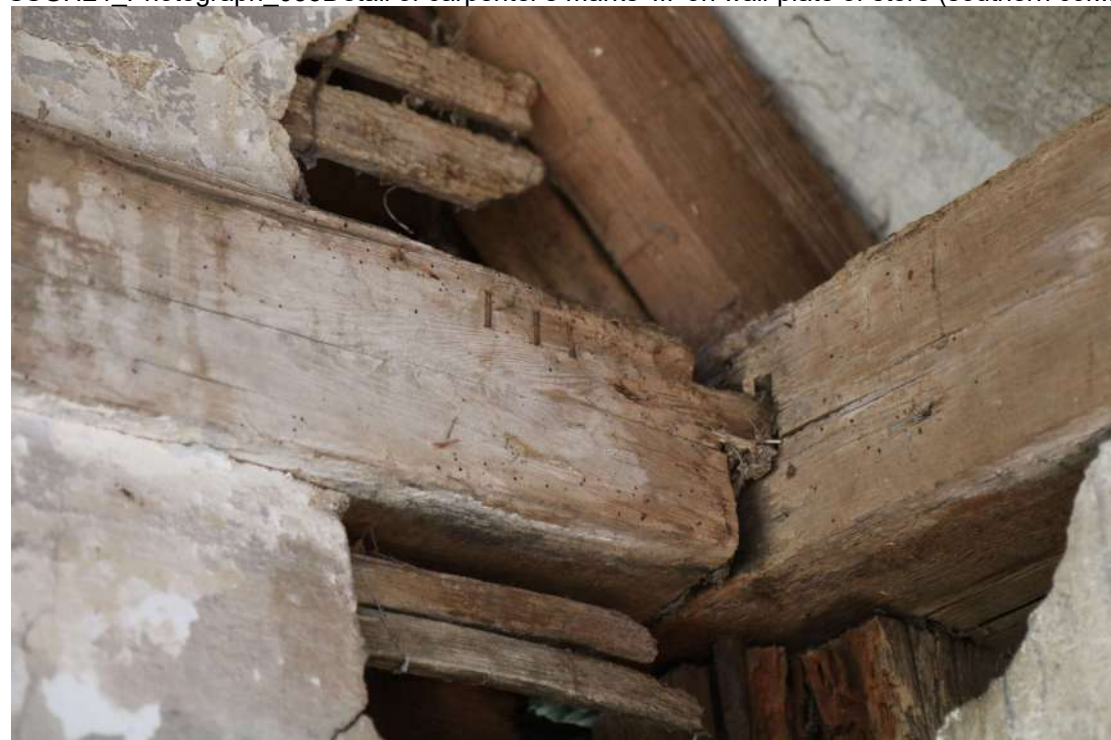
SSGH24_Photograph_035detail of Baltic timber mark on north-east purlin in roof of store. Ph...
