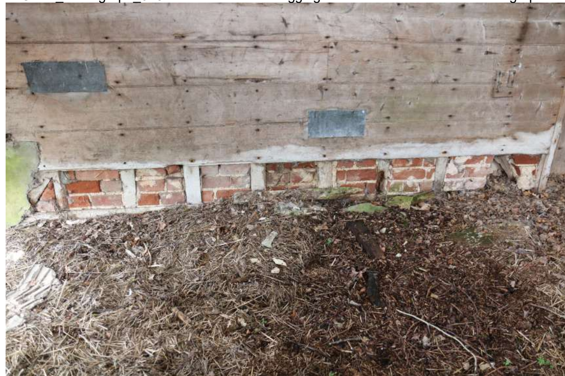
SSGH24_Photograph_048Detail of red brick nogging between store and barn. Photograph ta...
