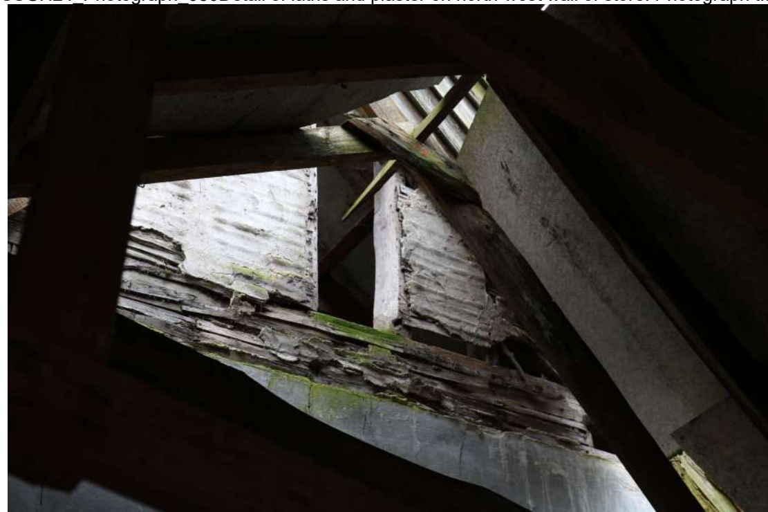
SSGH24 Photograph_032Detail of lath and plaster on south-west wall of store. Photograph t...
