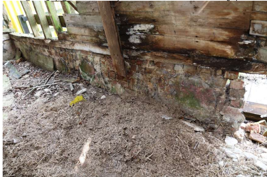
SSGH24 Photograph_055Detail of brick plinth on north-east wall of barn. Photograph taken f...
