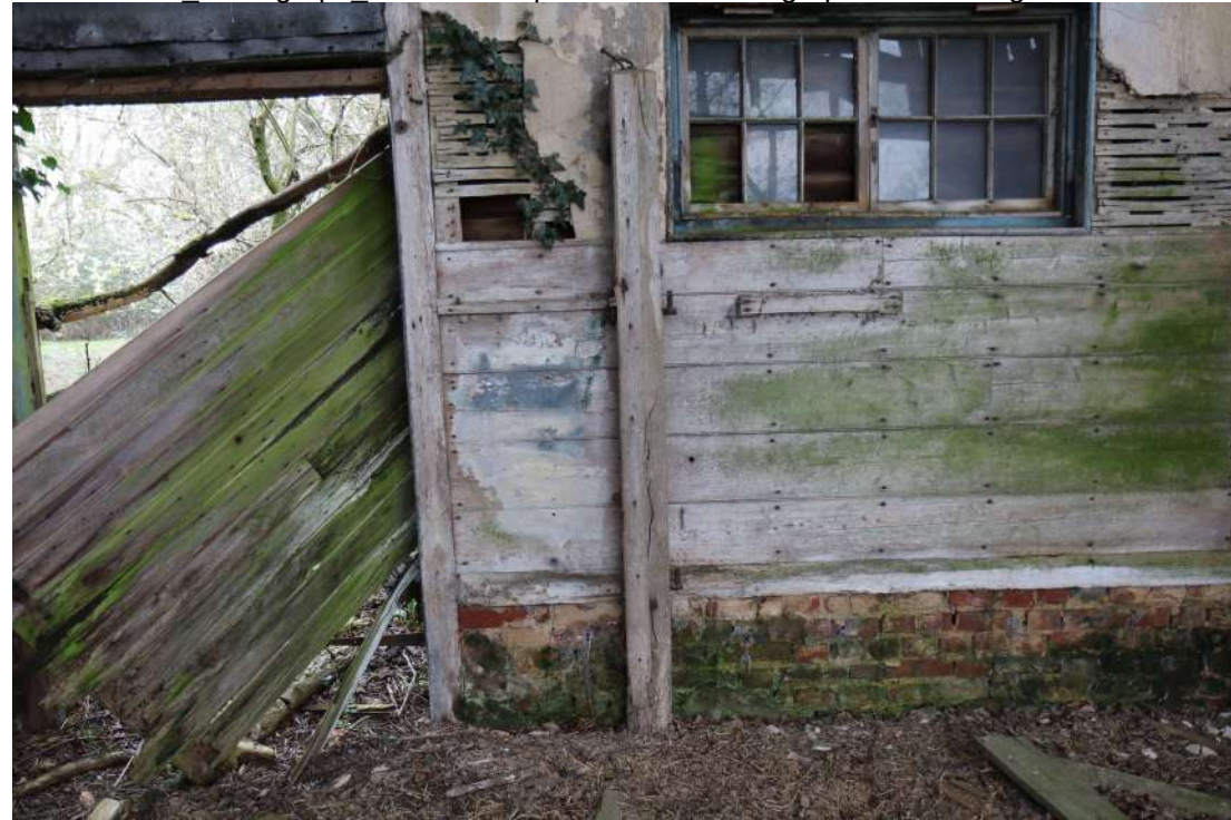
SSGH24 Photograph_052Detail of empty mortices in north-east sill-beam of barn. Photograp...
