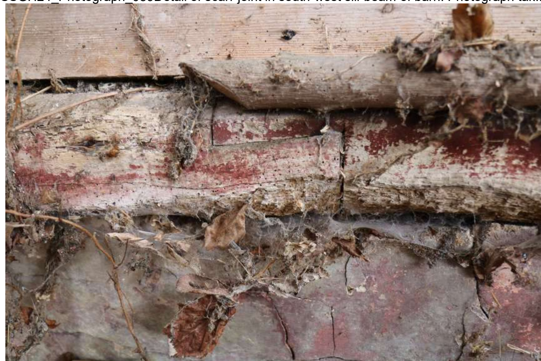
SSGH24_Photograph_059Detail of scarf-joint in south-west sill-beam of barn. Photograph tak...
