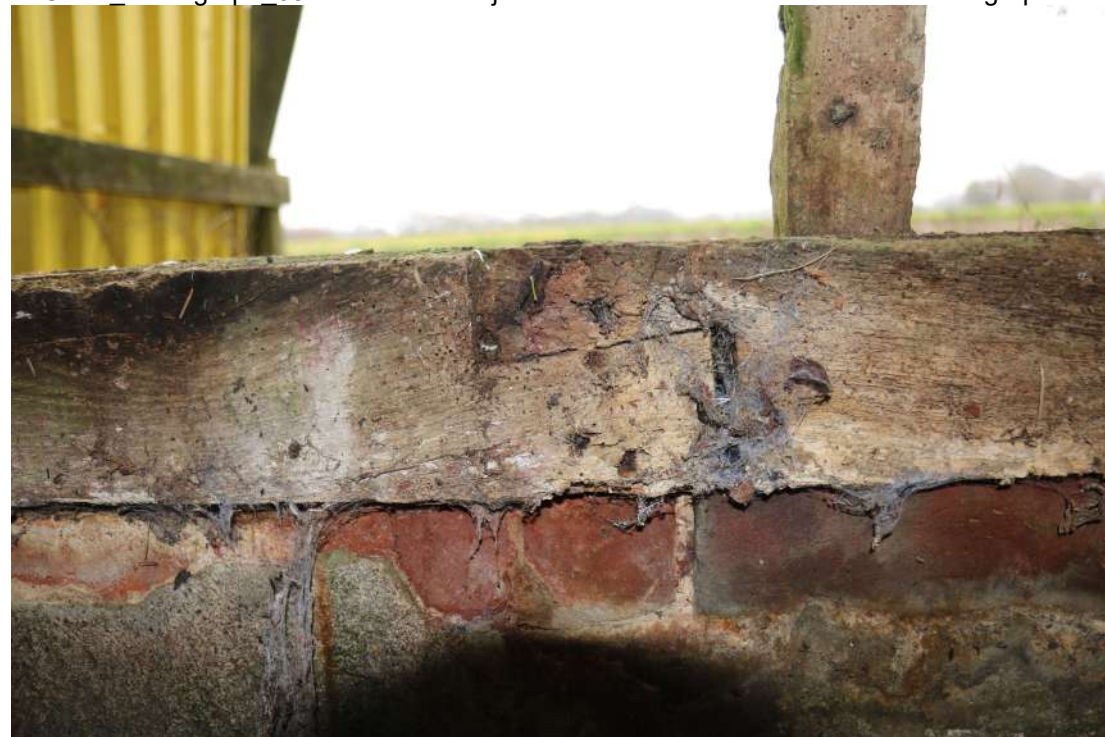
SSGH24 Photograph_051Detail of scarf-joint in north-east sill-beam of barn. Photograph tak...
