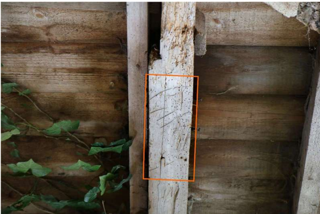
Photograph 15 Detail of Baltic timber mark on door post in south-west wall of barn. Photograph taken facing south-west.
