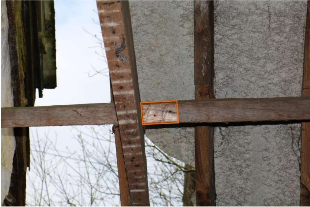
Photograph 20 Detail of Baltic timber mark on north-east purlin in roof of store. Photograph taken facing north-east.
