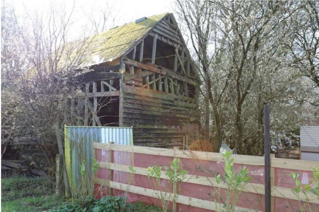
Photograph 8 North-west elevation. Photograph taken facing south-east.
