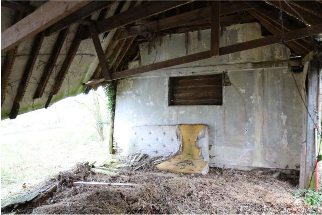
Photograph 18 Interior of store. Photograph taken facing east.
