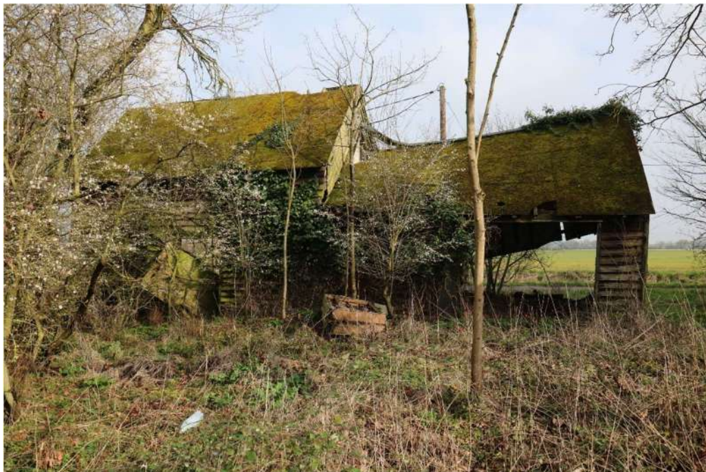
Photograph 1 South-west elevation. Photograph taken facing north north-east.
