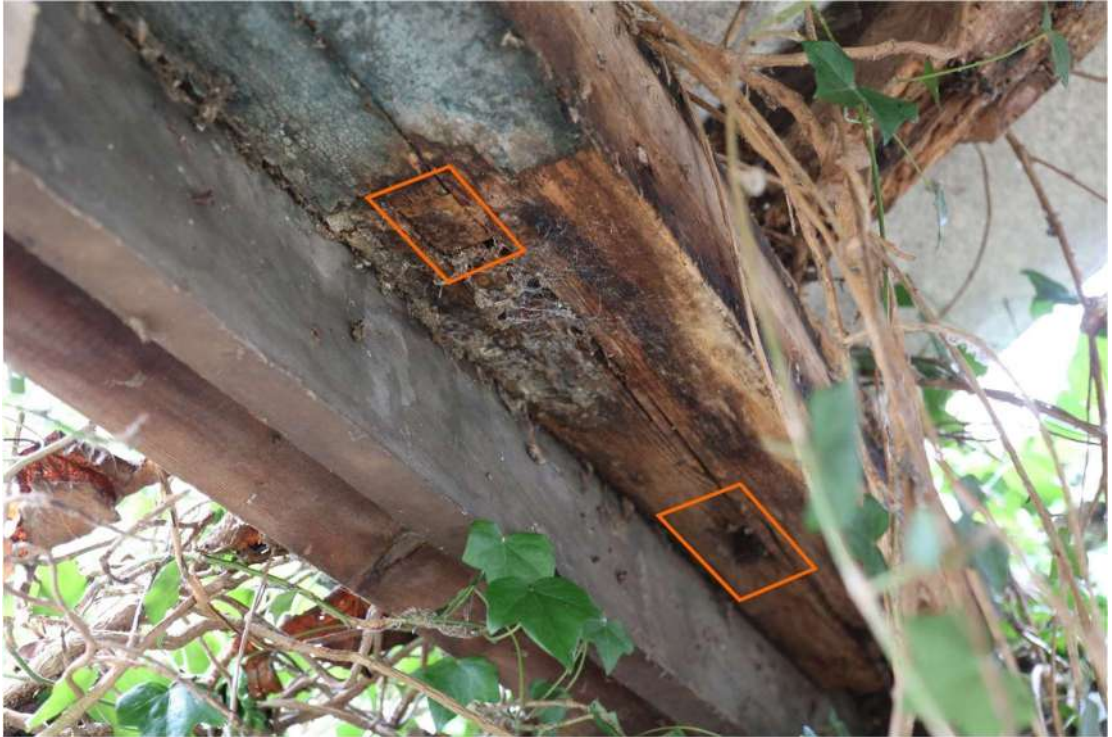
Photograph 24 Detail of empty mortices in wall-plate above south-western doorway. Photograph taken facing west.
