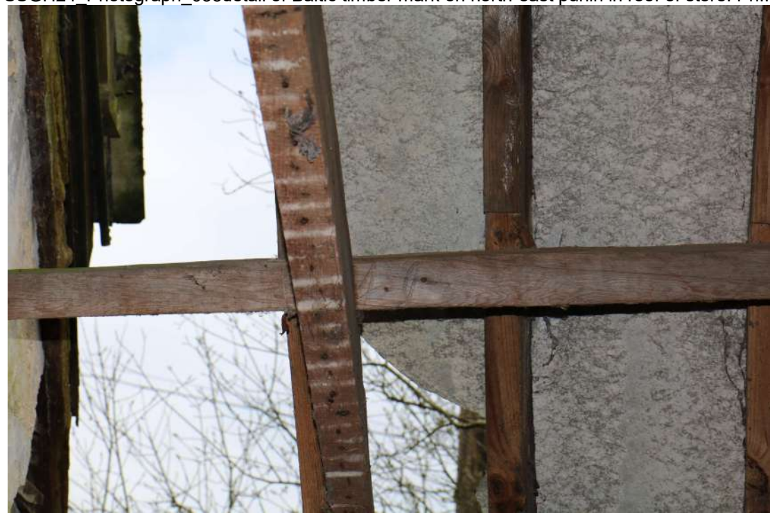
SSGH24_Photograph_035detail of Baltic timber mark on north-east purlin in roof of store. Ph...
