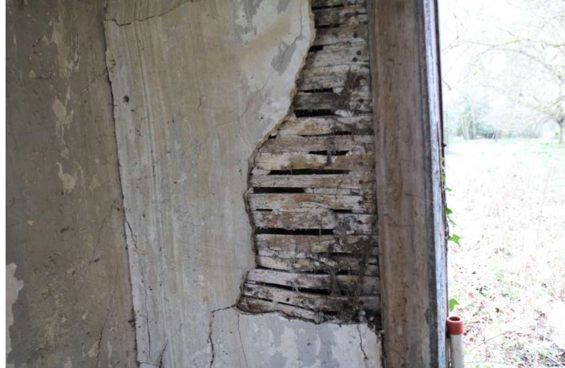
SSGH24 Photograph_032Detail of lath and plaster on south-west wall of store. Photograph t...
