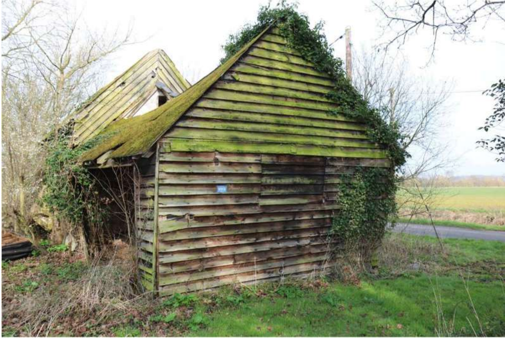
Photograph 6 South-east elevation. Photograph taken facing north.
