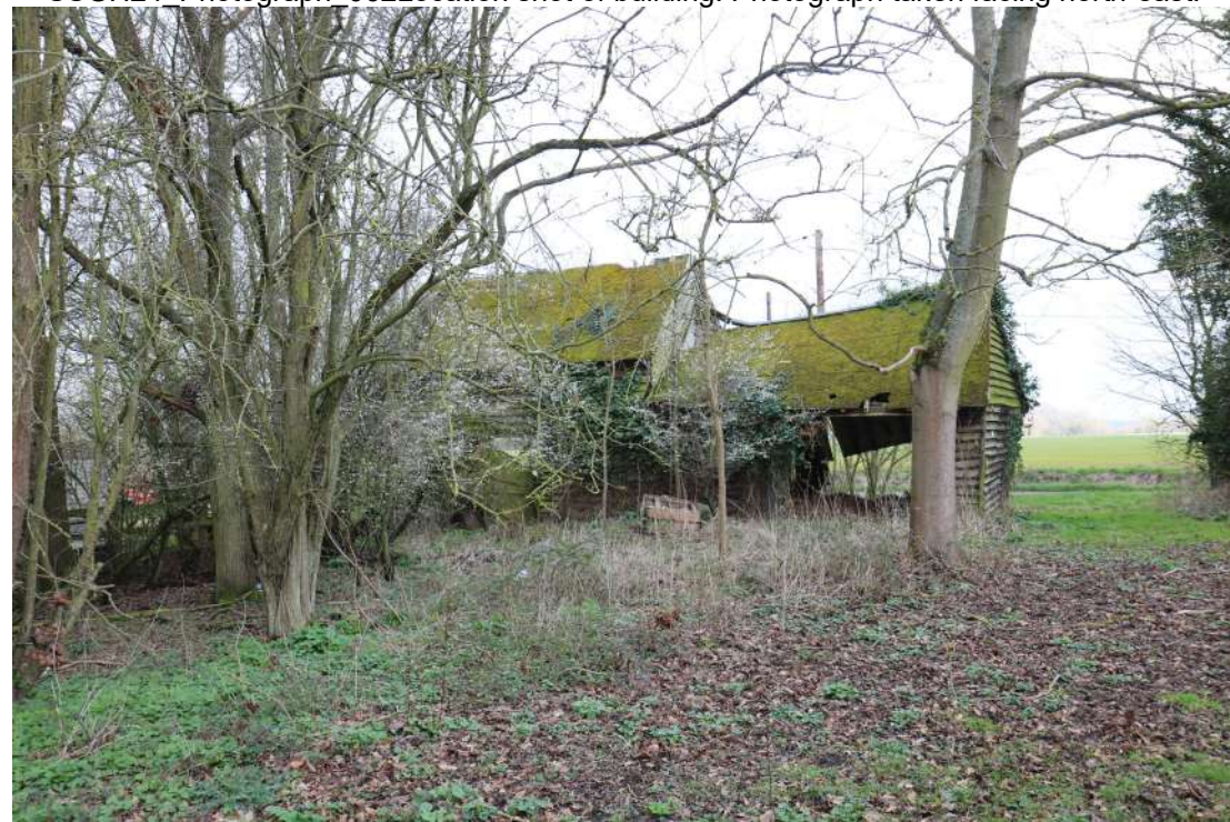
SSGH24_Photograph_062Location shot of building. Photograph taken facing north-east.
