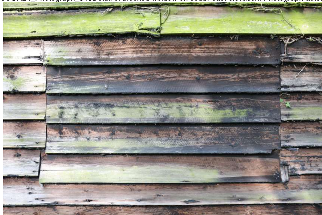
SSGH24_Photograph_015 Detail of blocked window on south-east elevation. Photograph take...
