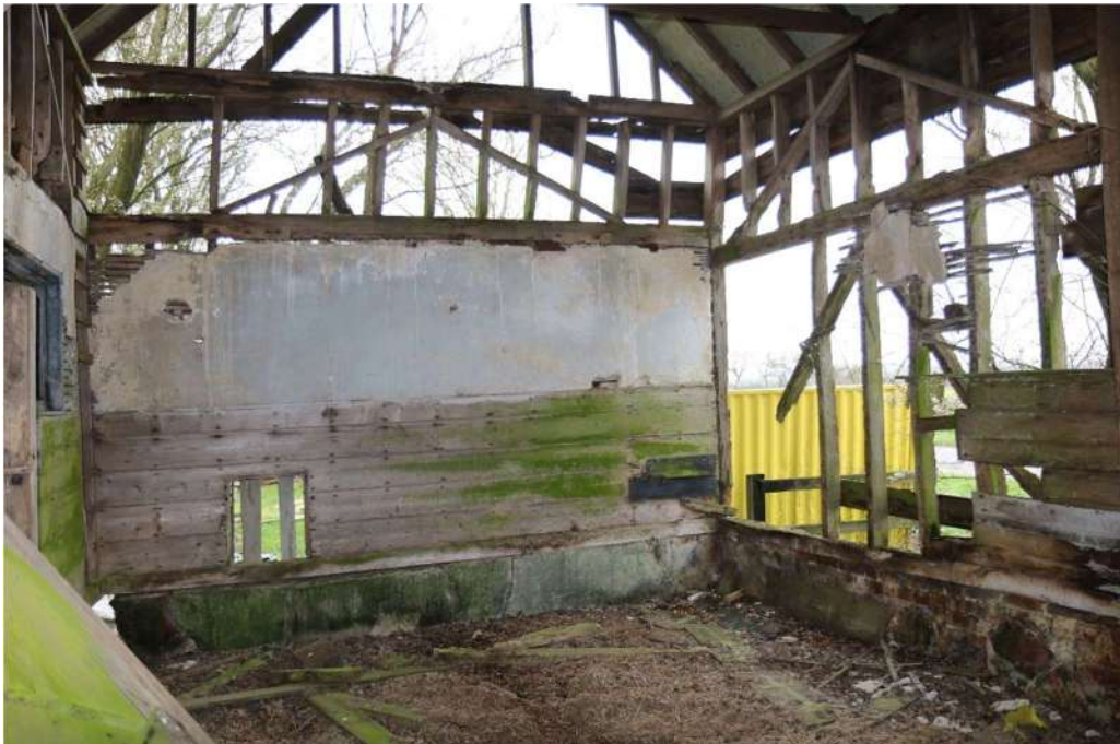
Photograph 11 Interior of barn. Photograph taken facing north.
