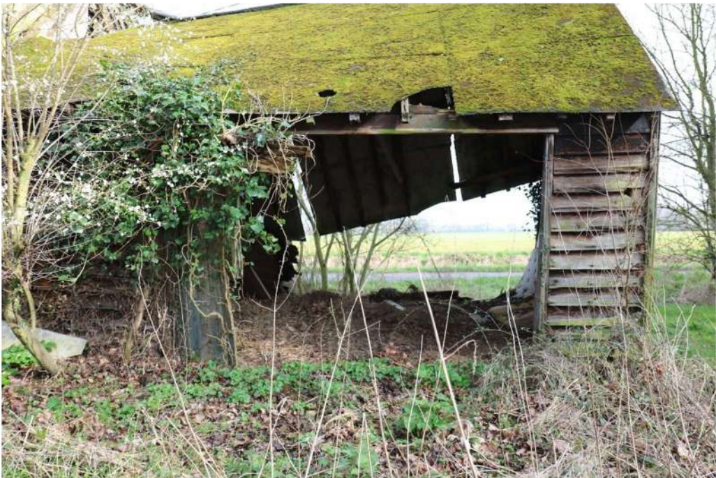
Photograph 5 Detail of double doors on south-west elevation. Photograph taken facing north-east.
