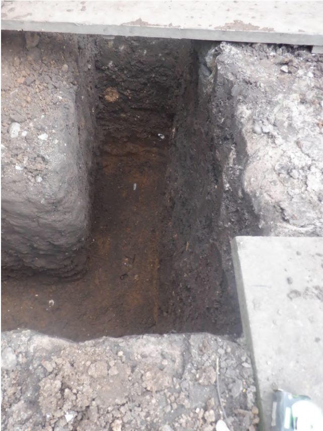
Photograph 3 Foundation trench, looking east.
