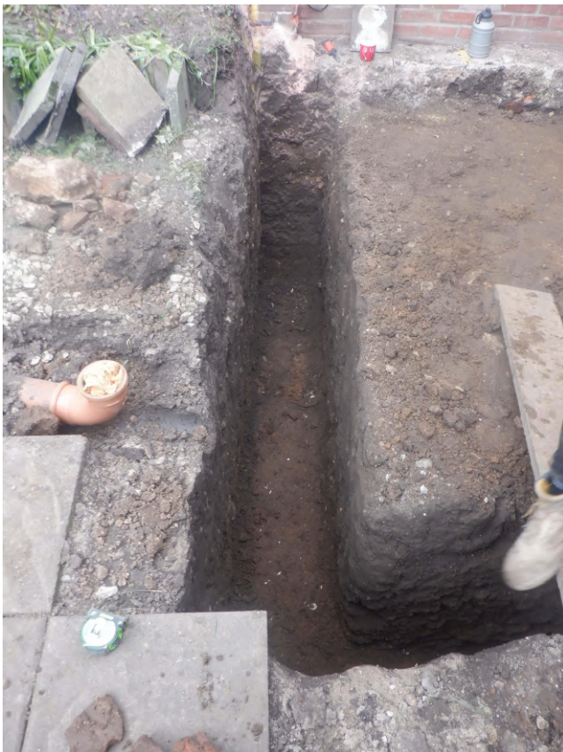
Photograph 2 Foundation trench, looking north.
