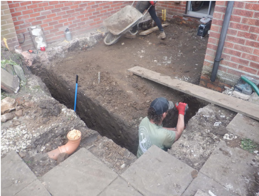
Photograph 1 Excavation of the foundation trenches, looking north-east.
