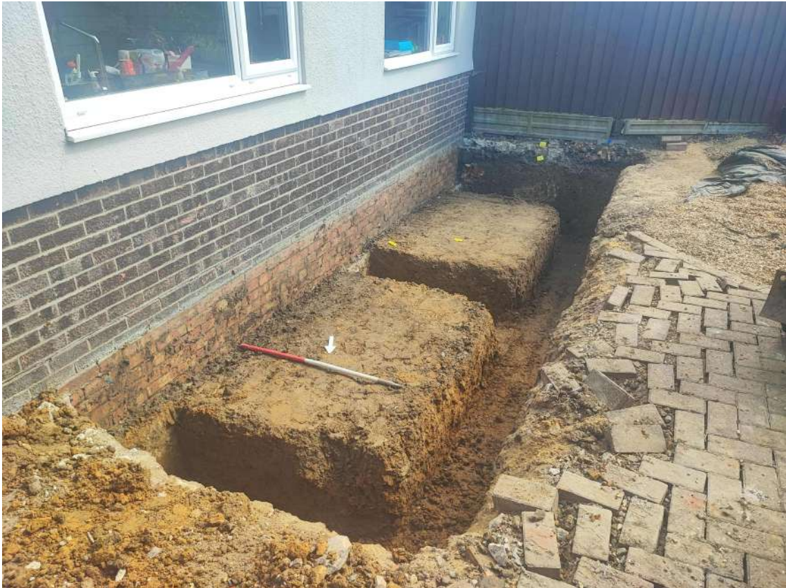
Photograph 1 General shot of completed trenches, looking south-east.
