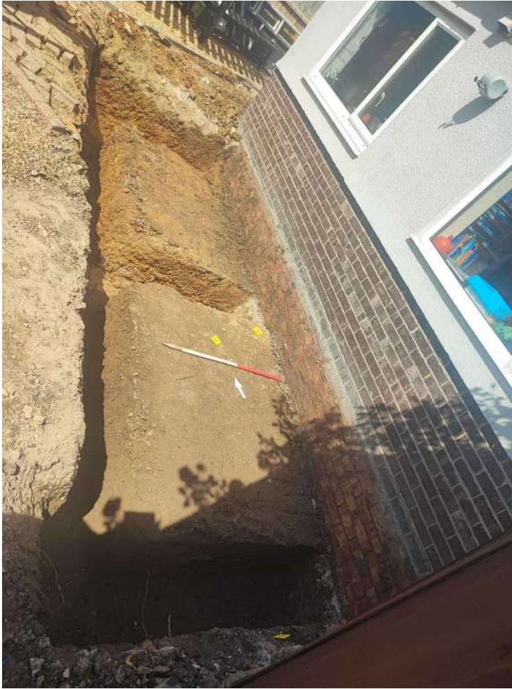
Photograph 2 General shot of completed trenches, looking north-east
