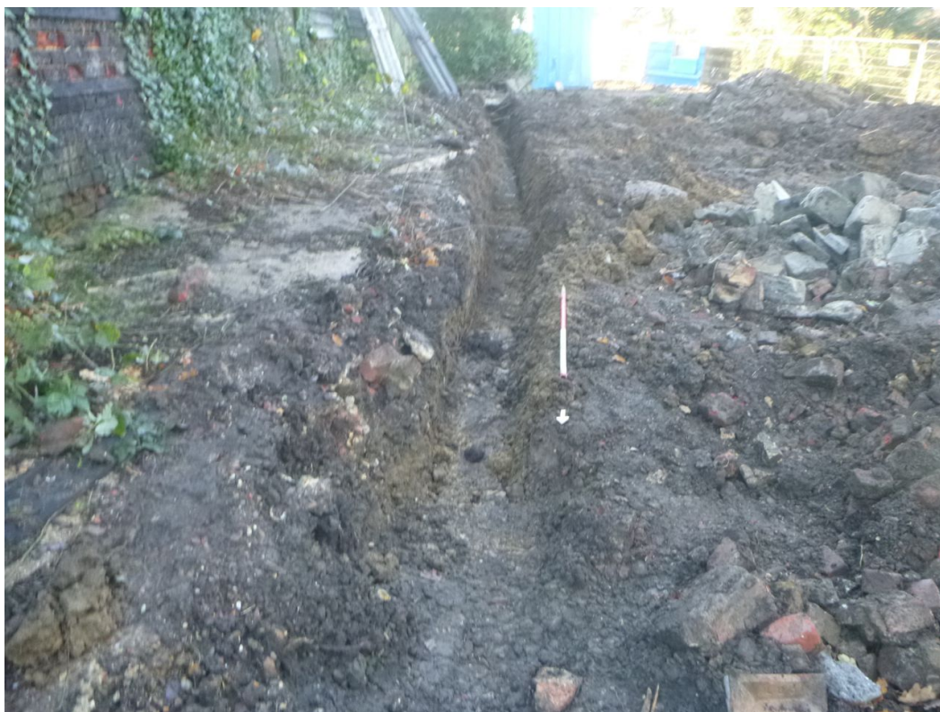
Photograph 1 Drainage trench, looking south-south-west.
