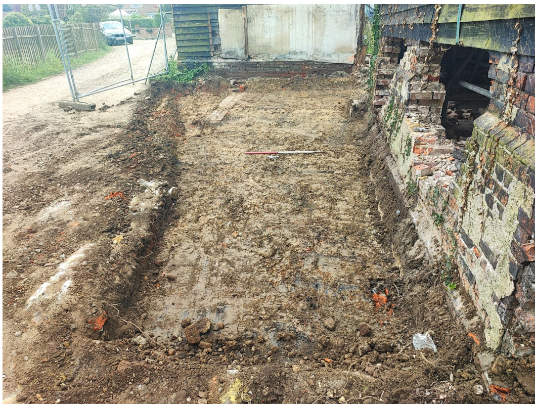
Photograph 2 Stripped area, looking east-south-east.
