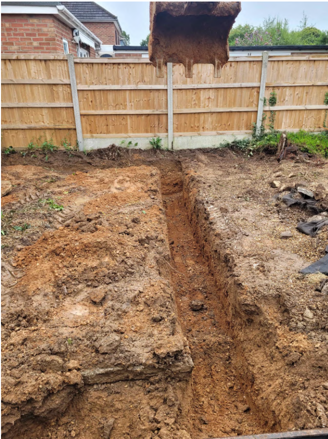
Photograph 2 Foundation trench, looking south-east.
