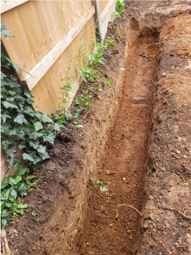
Photograph 1 Foundation trench, looking south-south-west.
