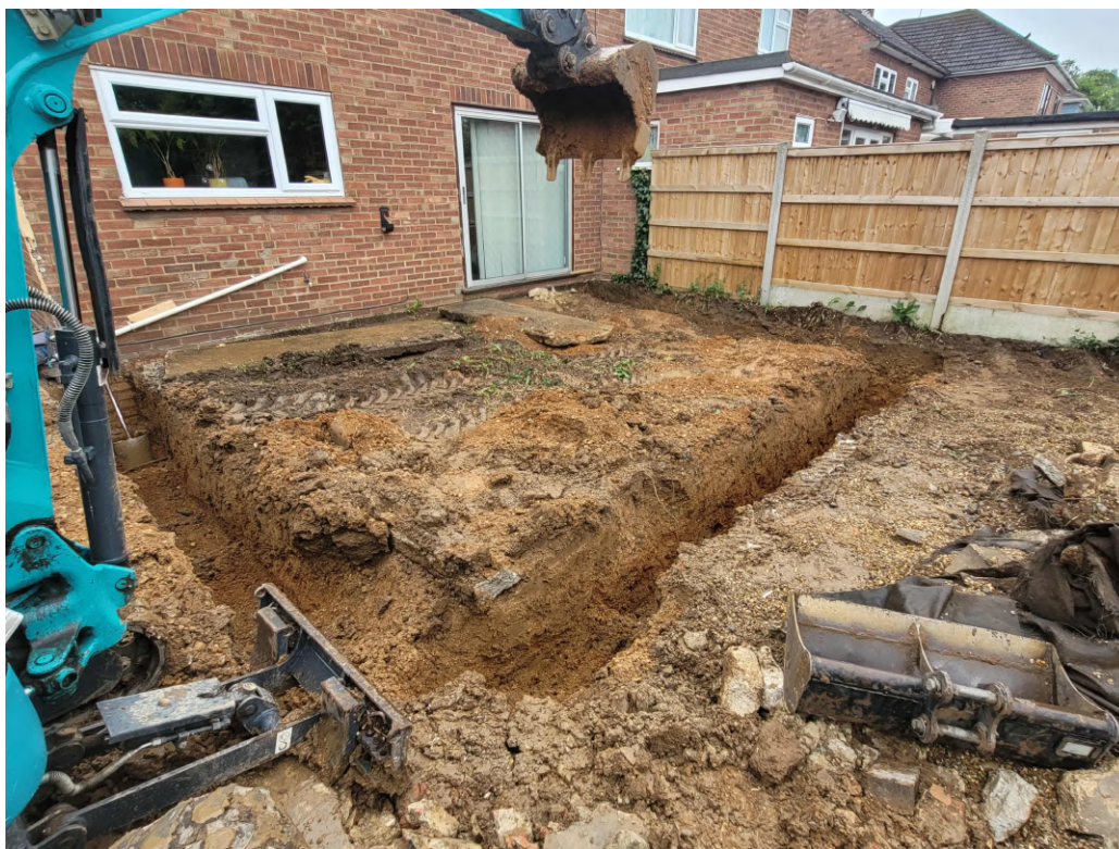
Photograph 3 Foundation trench, looking south-east.
