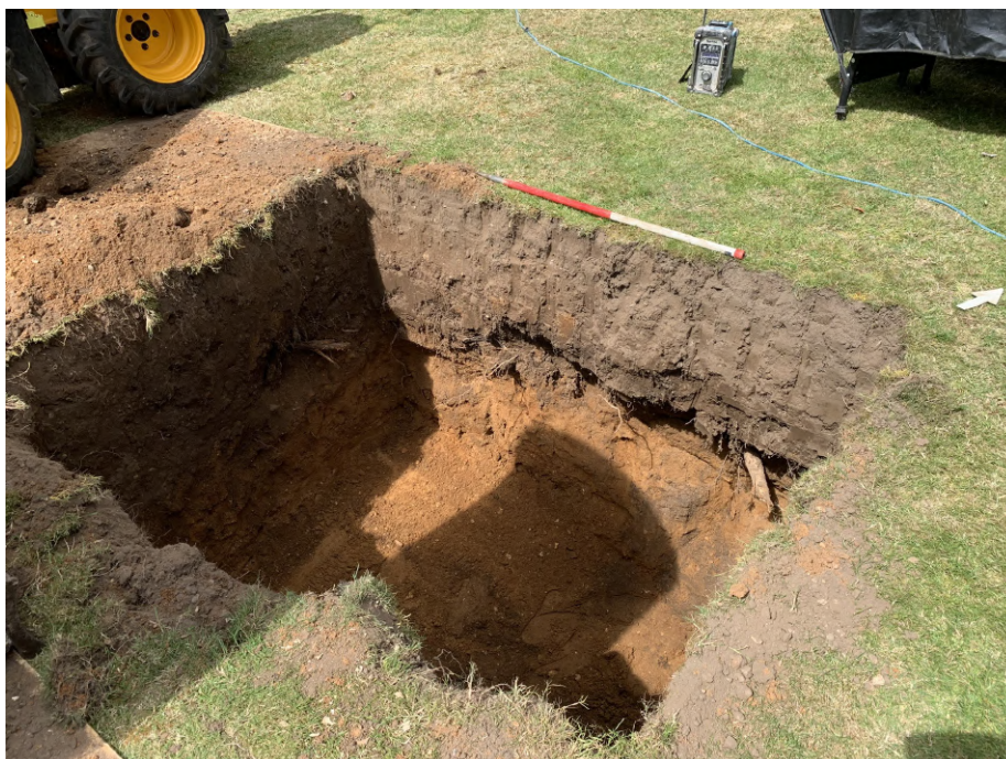
Photograph 1 Soakaway, looking north-west.
