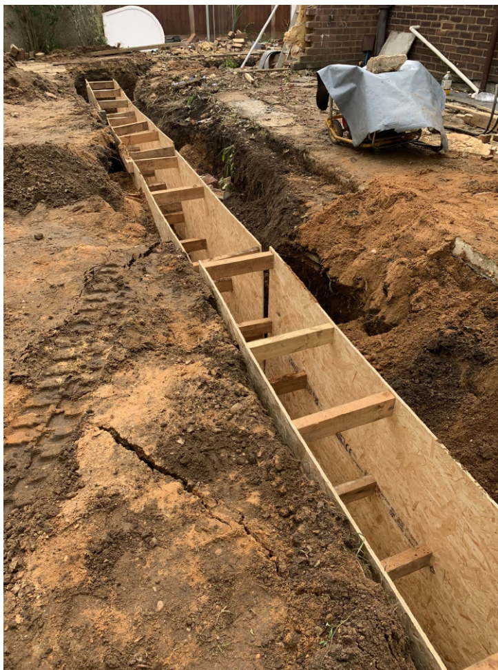
Photograph 3 Trench shuttering, looking north.
