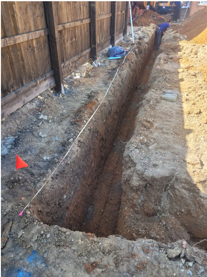
Photograph 1 Foundation trench, looking south-west.
