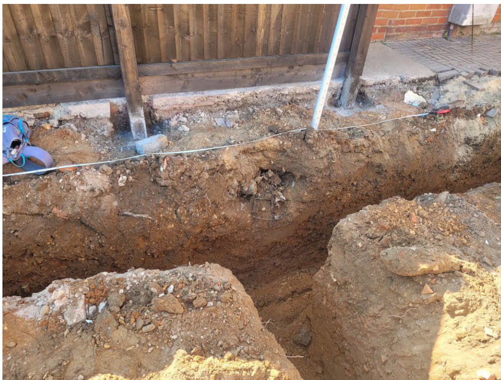
Photograph 3 Foundation trench and F2, looking south-east.
