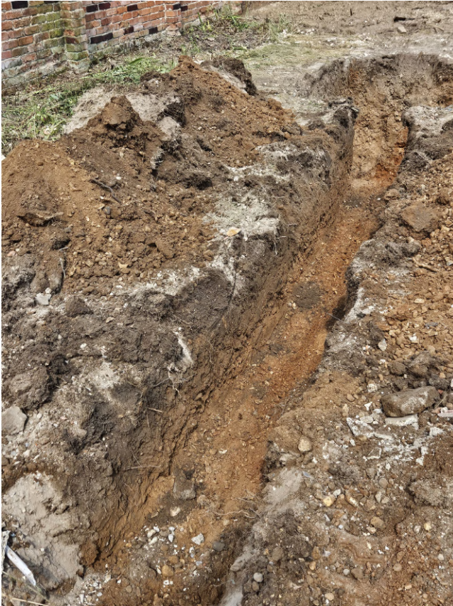
Photograph 4 Service trench leading to soakaway, looking north-east.
