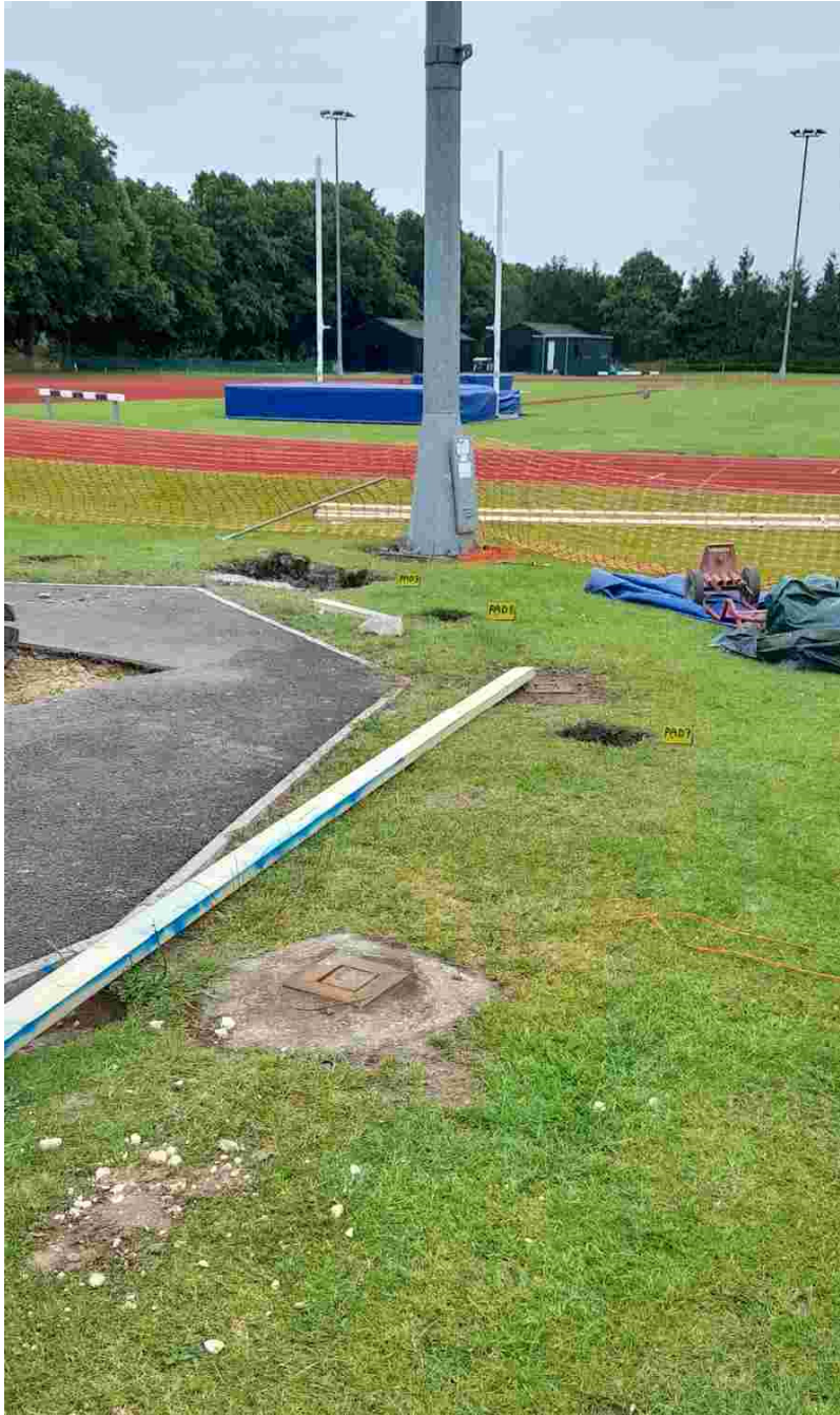
Photograph 2 Pads 7-8 (foreground) Pad 3 (background), looking south/south-west.
