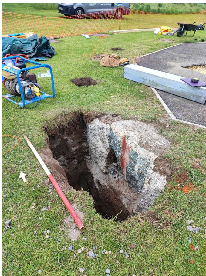
Photograph 4 Pad 3 fully excavated, looking north/north-east.
