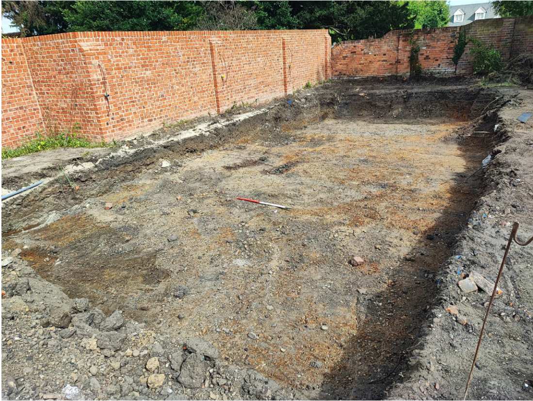
Photograph 4 Stripped footprint of the swimming pool, looking east.
