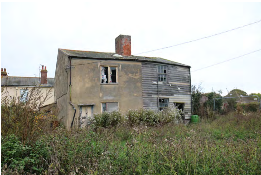
EEX60394_PhotoGraph_023 Eastern elevation of semi-detached houses. Photograph taken facing north-west.
