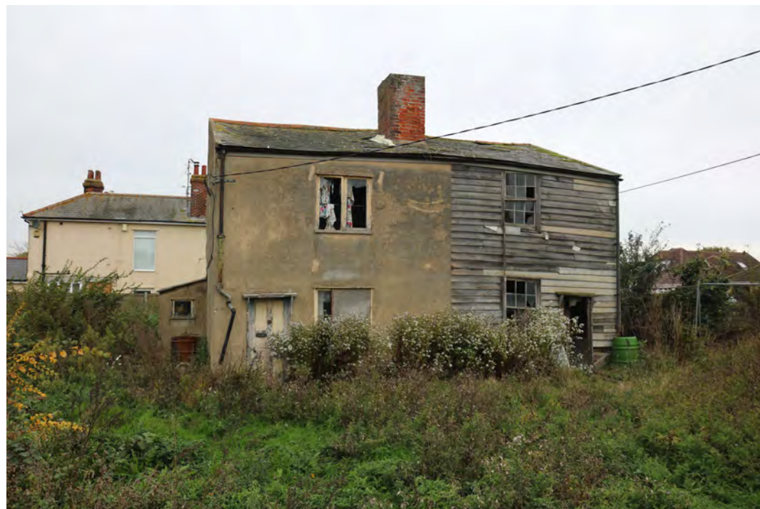
EEX60394_PhotoGraph_024 Eastern elevation of semi-detached houses. Photograph taken facing north-west.
