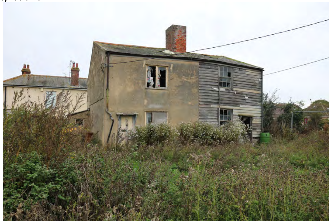
EEX60394_PhotoGraph_022 Eastern elevation of semi-detached houses. Photograph taken facing north-west.
