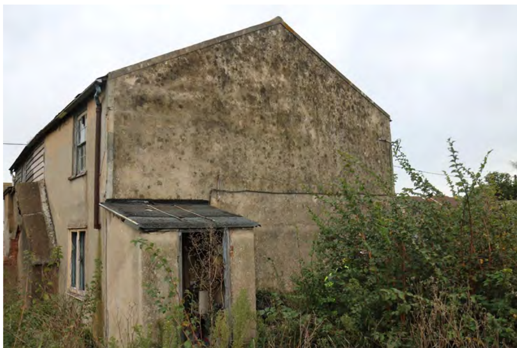
Photograph 5 Southern elevation of building A. Photograph taken facing north-east.
