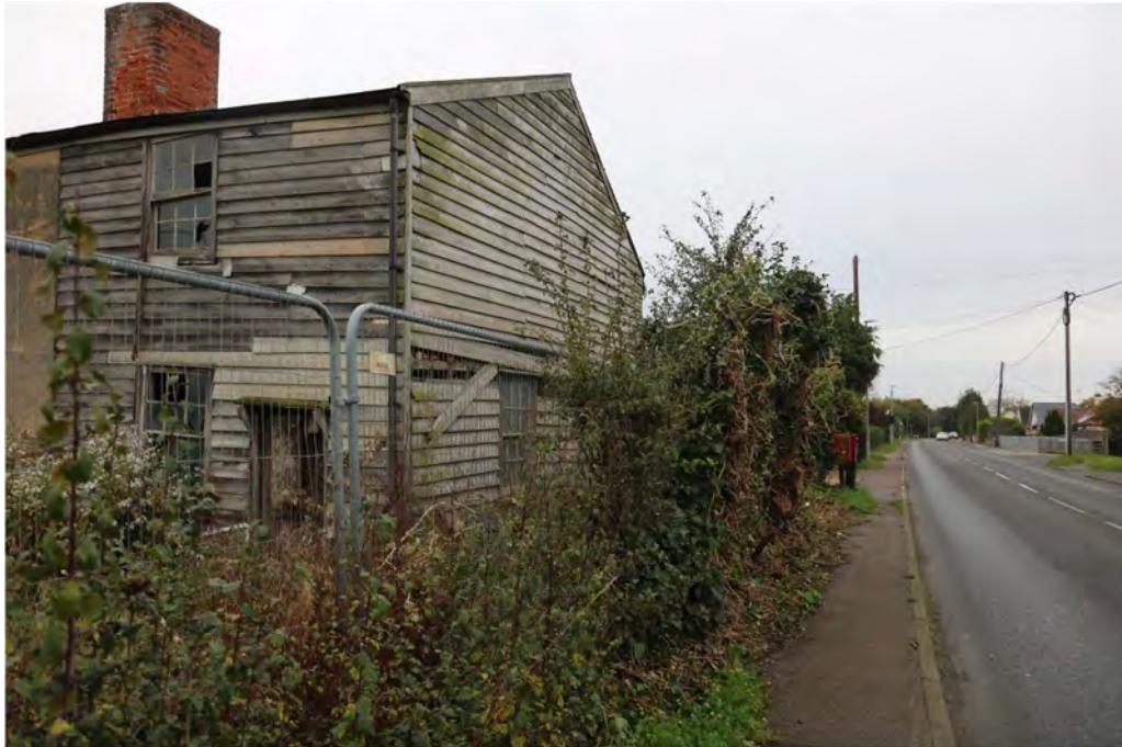
Photograph 8 Eastern and northern elevation of building B. Photograph taken facing south-west.
