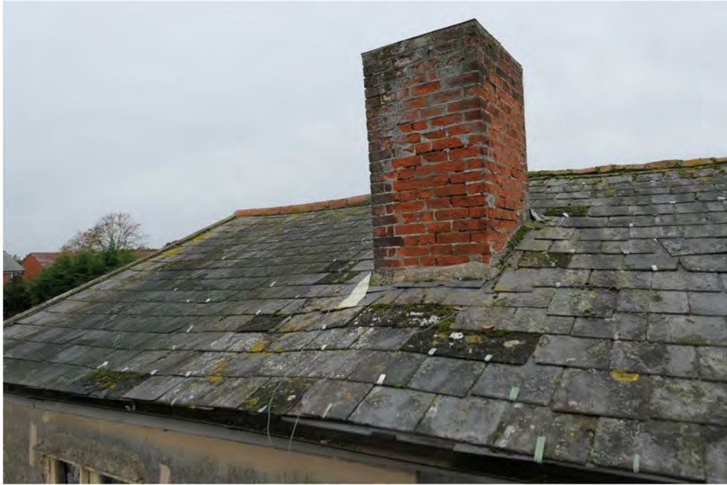
Photograph 2 Detail of red brick chimney. Photograph taken facing south-west.
