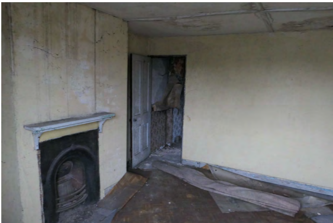
EEX60394_PhotoGraph_039 First floor window on western elevation of building 2. Photograph taken facing east.
