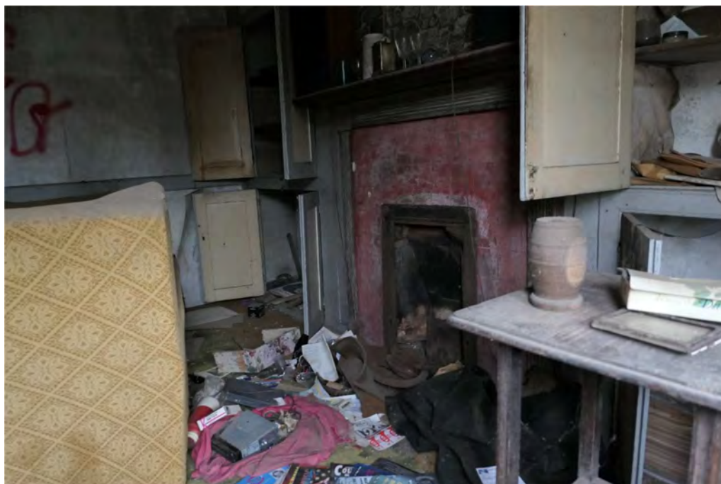
Photograph 11 Fireplace in room A2, building A. Photograph taken facing north-west.
