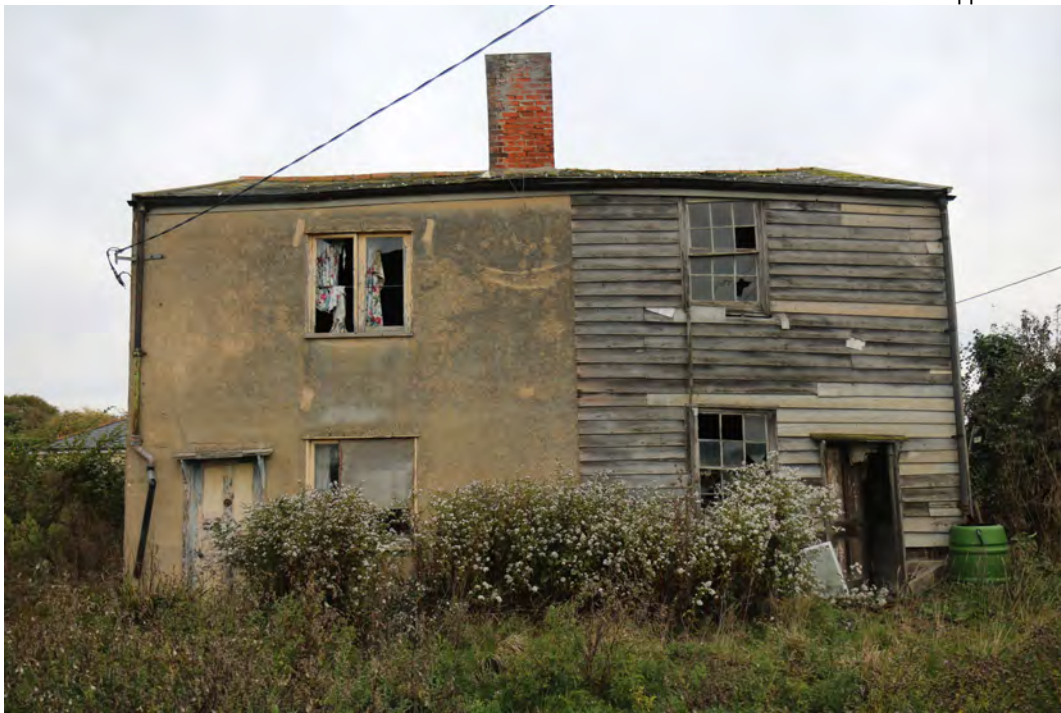
EEX60394_PhotoGraph_001 Eastern elevation of semi-detached houses. Photograph taken facing west.
