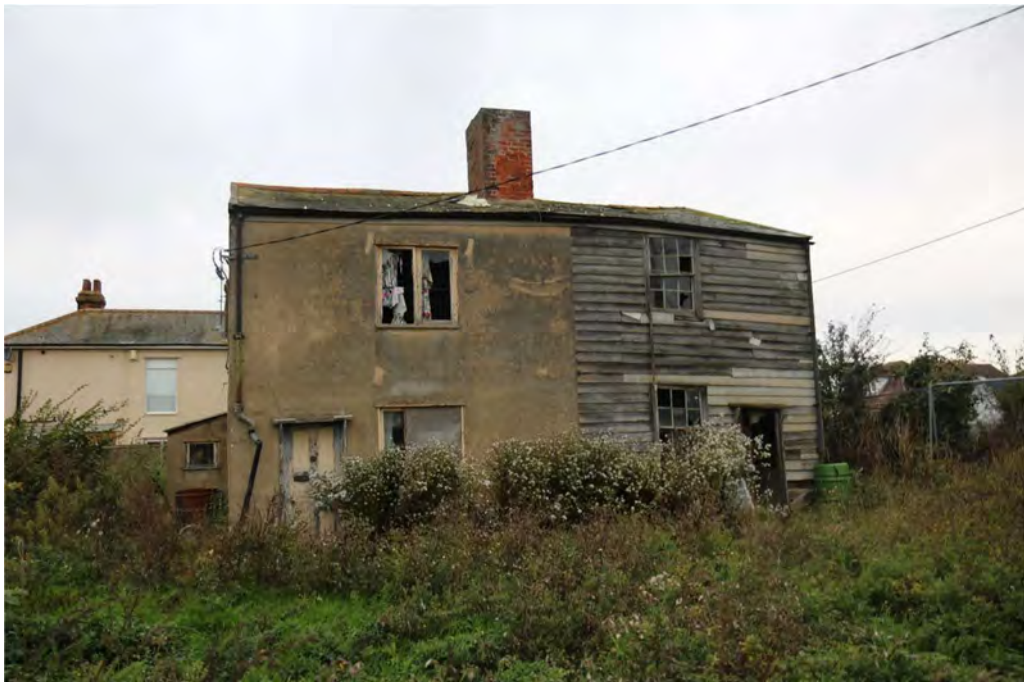
Photograph 1 Eastern elevation of semi-detached cottages with building A to the left. Photograph taken facing west.
