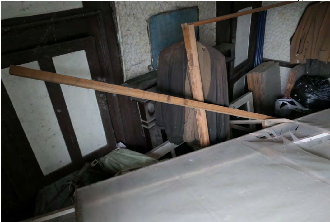
EEX60394_PhotoGraph_029 Interior of room 2 in building B. Photograph taken facing west south-west
