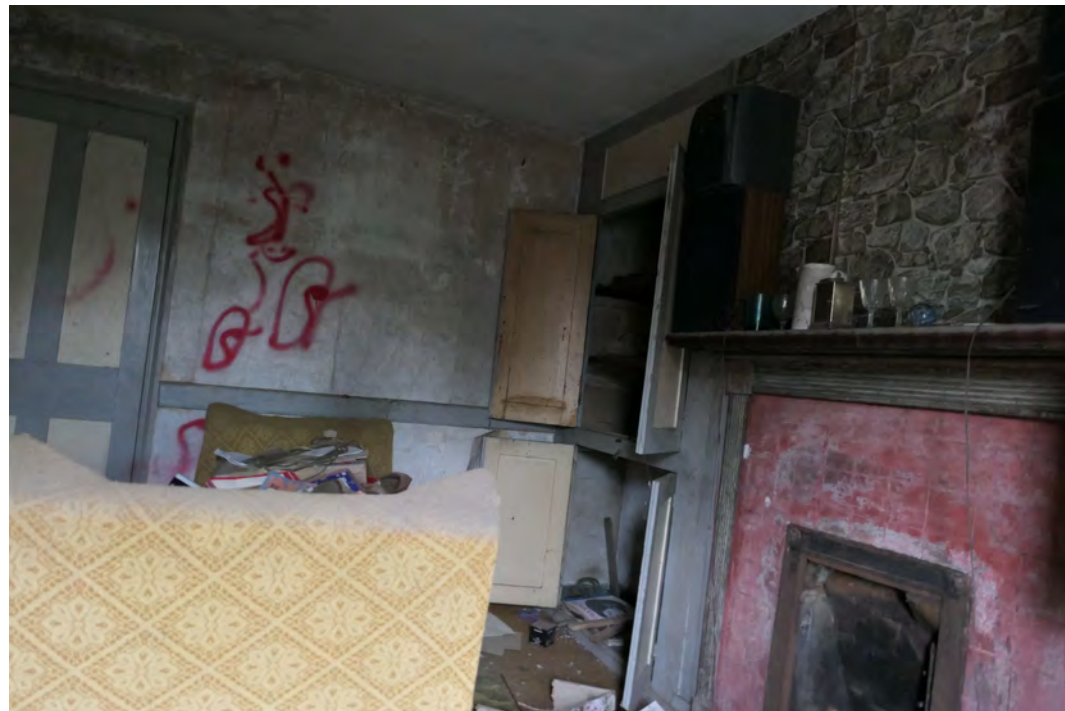
EEX60394_PhotoGraph_044 Interior of room 2 on the ground floor in building A. Photograph taken facing north-west.
