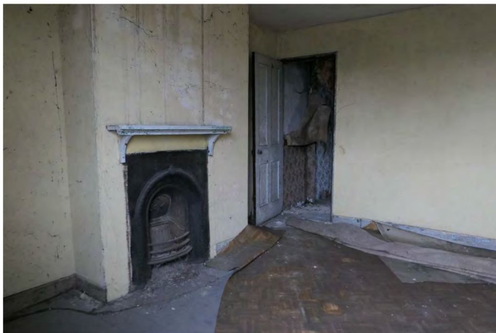
Photograph 17 Interior of room 4, building 2, showing the fireplace. Photograph taken facing south-west.
