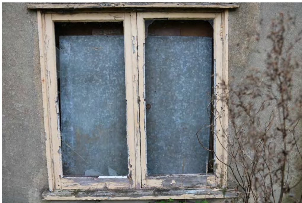
Photograph 4 Ground floor casement window on western elevation of building A. Photograph taken facing east.
