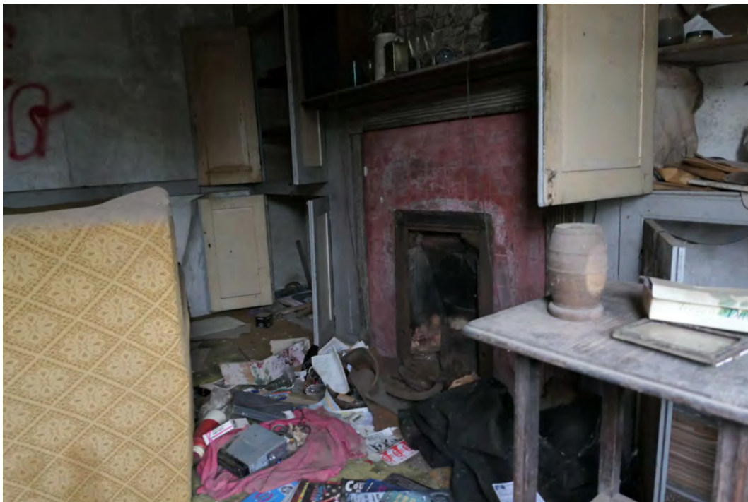
EEX60394_PhotoGraph_043 First floor window on western elevation of building 1. Photograph taken facing east.
