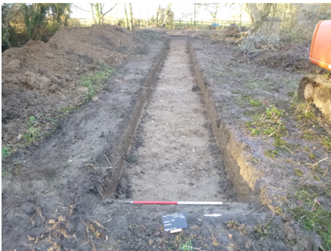
Photograph 2 Trench 2, looking west.
