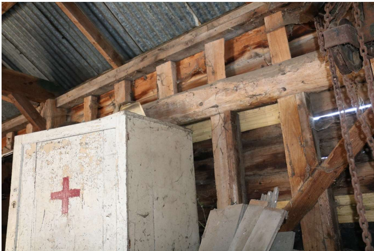
Photograph 36 Detail of pegged studs in north-eastern wall of bay 2 of threshing barn B. Photograph taken facing north.
