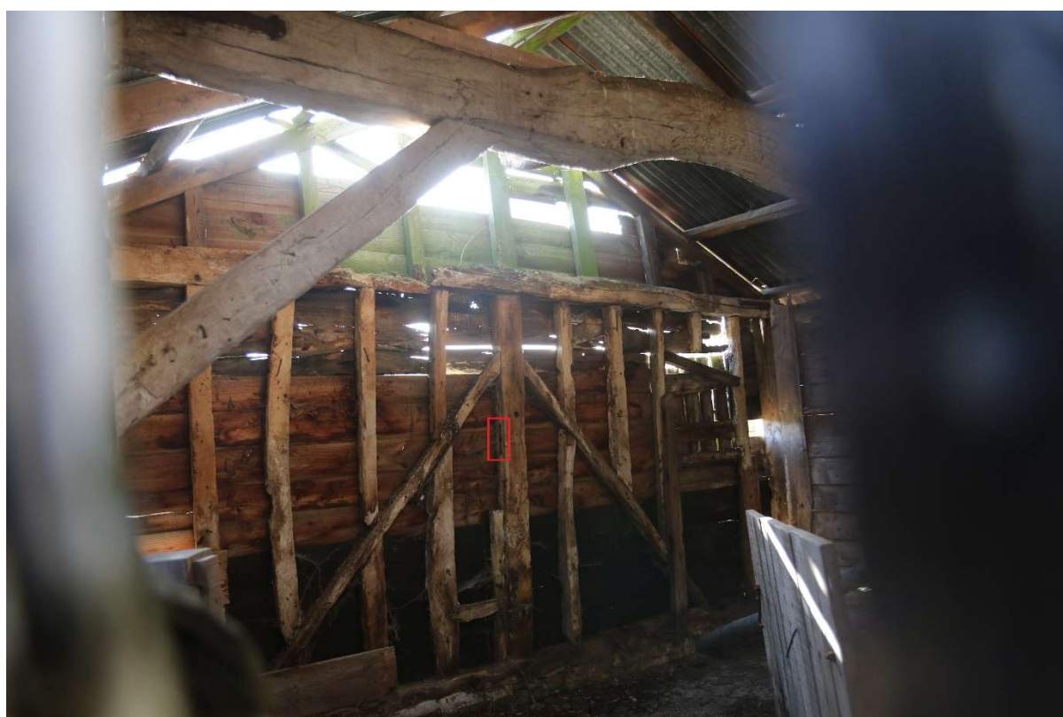
Photograph 51 Detail of reused centre-post of south-western wall of stable. Photograph taken facing south-west. (Empty mortice highlighted with red box)
