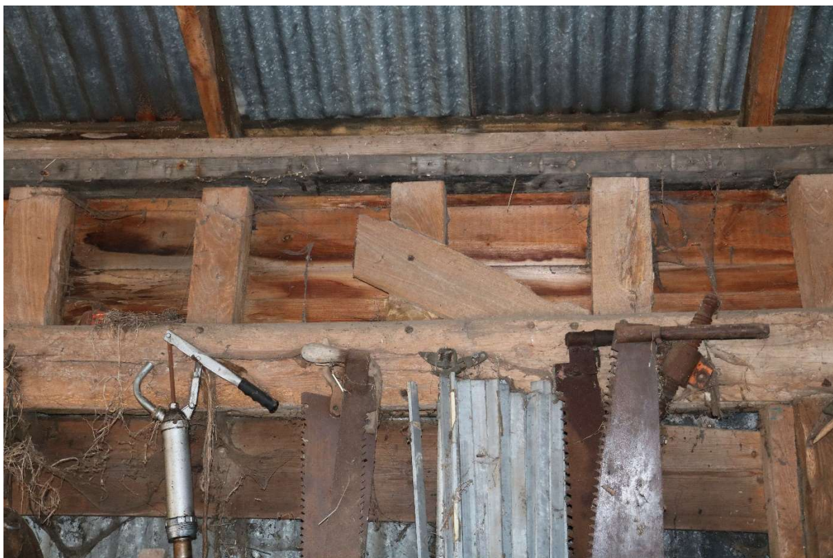
Photograph 37 Detail of reduced tension brace in bay 3 of threshing barn B. Photograph taken facing north-east.
