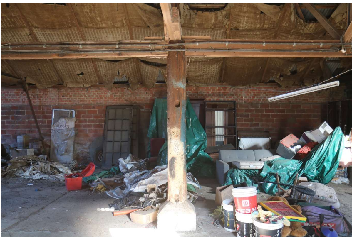
Photograph 47 Detail of reused centre-post of linking shed. Photograph taken facing north-east.
