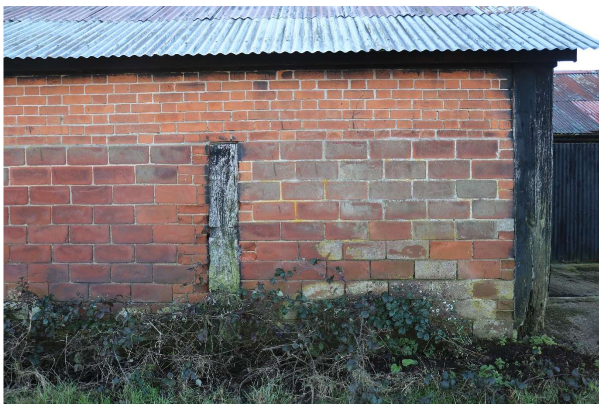
Photograph 11 Detail of reused timber post on north-east elevation of linking shed. Photograph taken facing south south-east.
