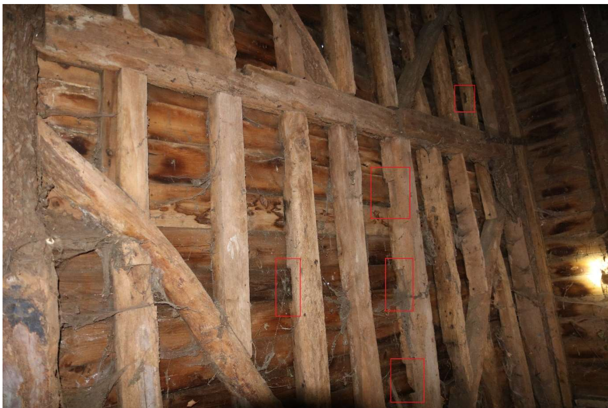
Photograph 28 Detail of reused studs in north-western wall of bay 5 of threshing barn A. Photograph taken facing north-west. (Empty mortices highlighted with red boxes)
