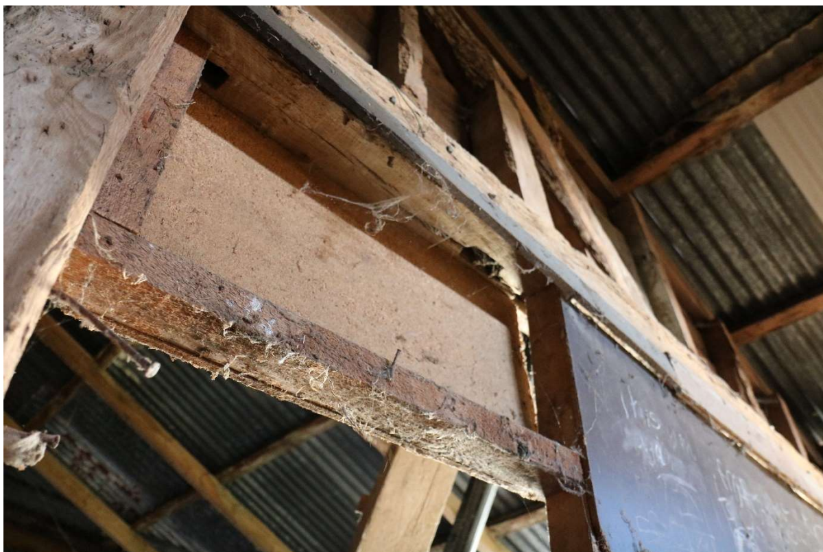
Photograph 31 Detail of empty mortices in girthing beam of north-western wall of midstrey of threshing barn A. Photograph taken facing north-east.
