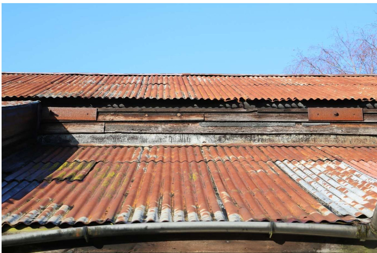
Photograph 7 Detail of anchor plates on south-east elevation of threshing barn A. Photograph taken facing west north-west.
