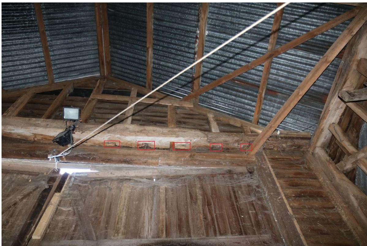
Photograph 29 Detail of empty mortices (highlighted with red boxes) in wall-plate in north-eastern wall of bay 5 of threshing barn A. Photograph taken facing north.
