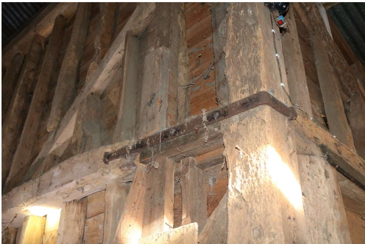
Photograph 24 Detail of iron strap on girding-beam and intermediate post of bay 4 of threshing barn A. Photograph taken facing east.
