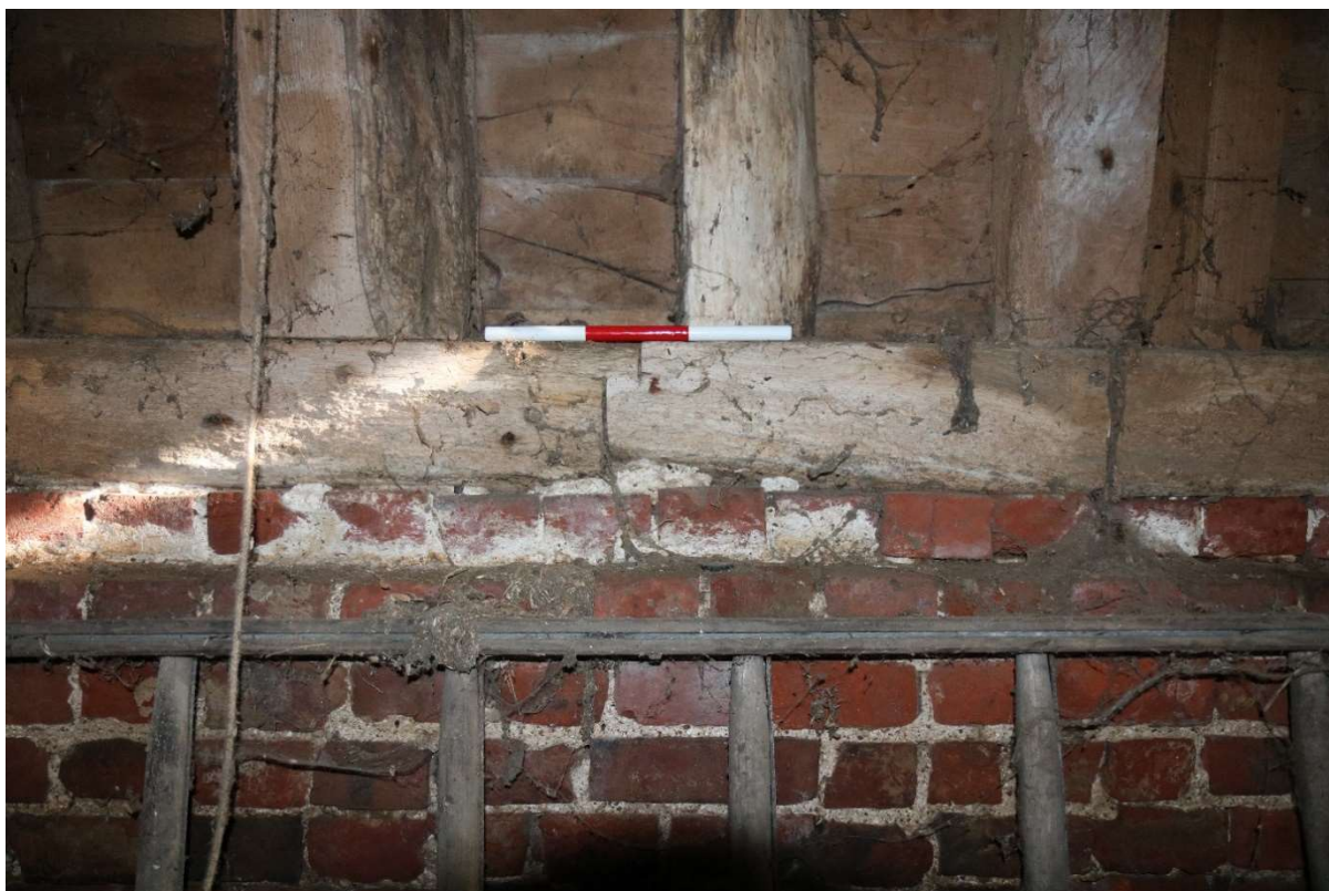
Photograph 23 Detail of scarf joint in sill-beam of south-eastern wall of bay 4 of threshing barn A. Photograph taken facing east south-east.
