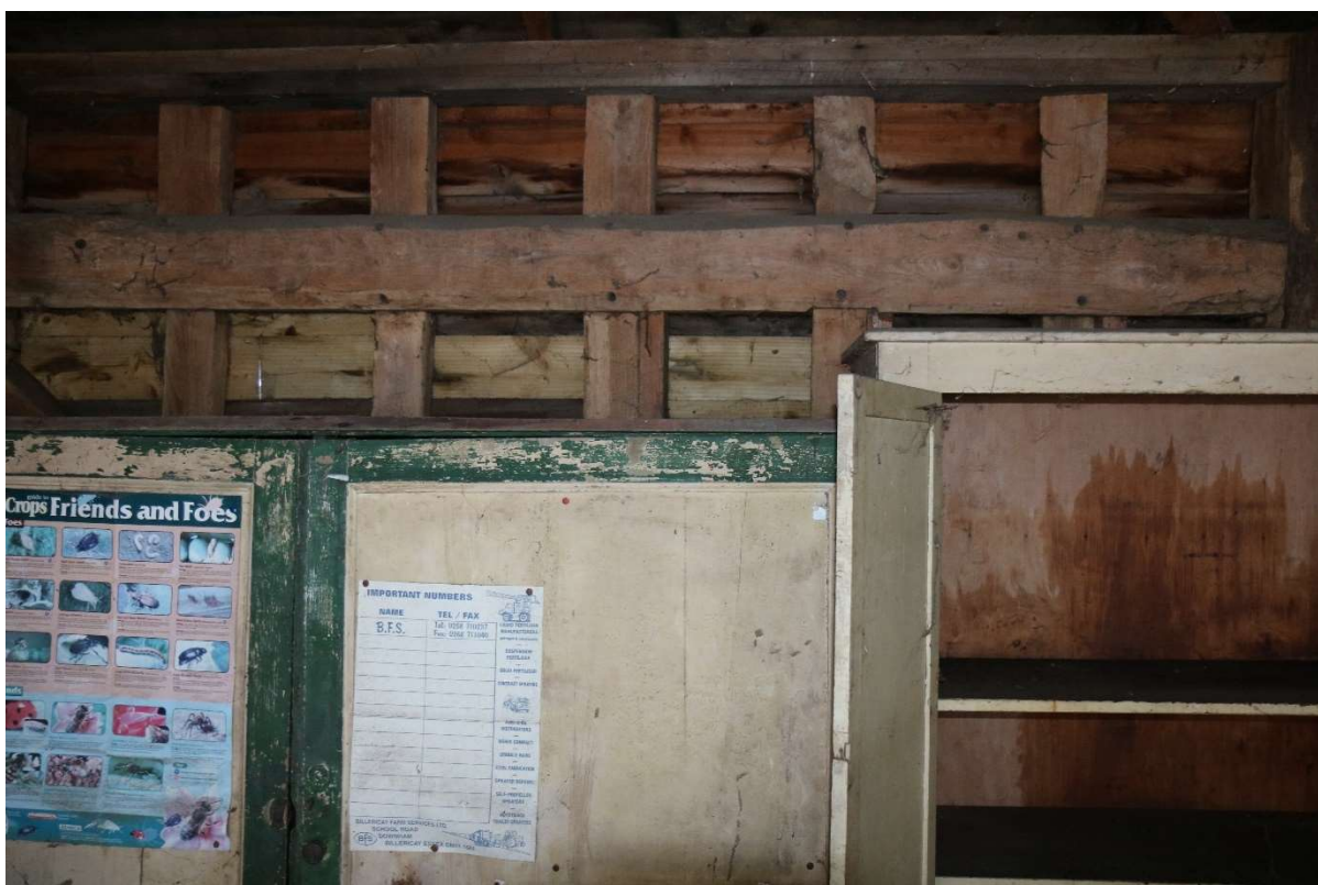
Photograph 35 Detail of pegged studs in the north-eastern wall of bay 1 of threshing barn B. Photograph taken facing north-east.
