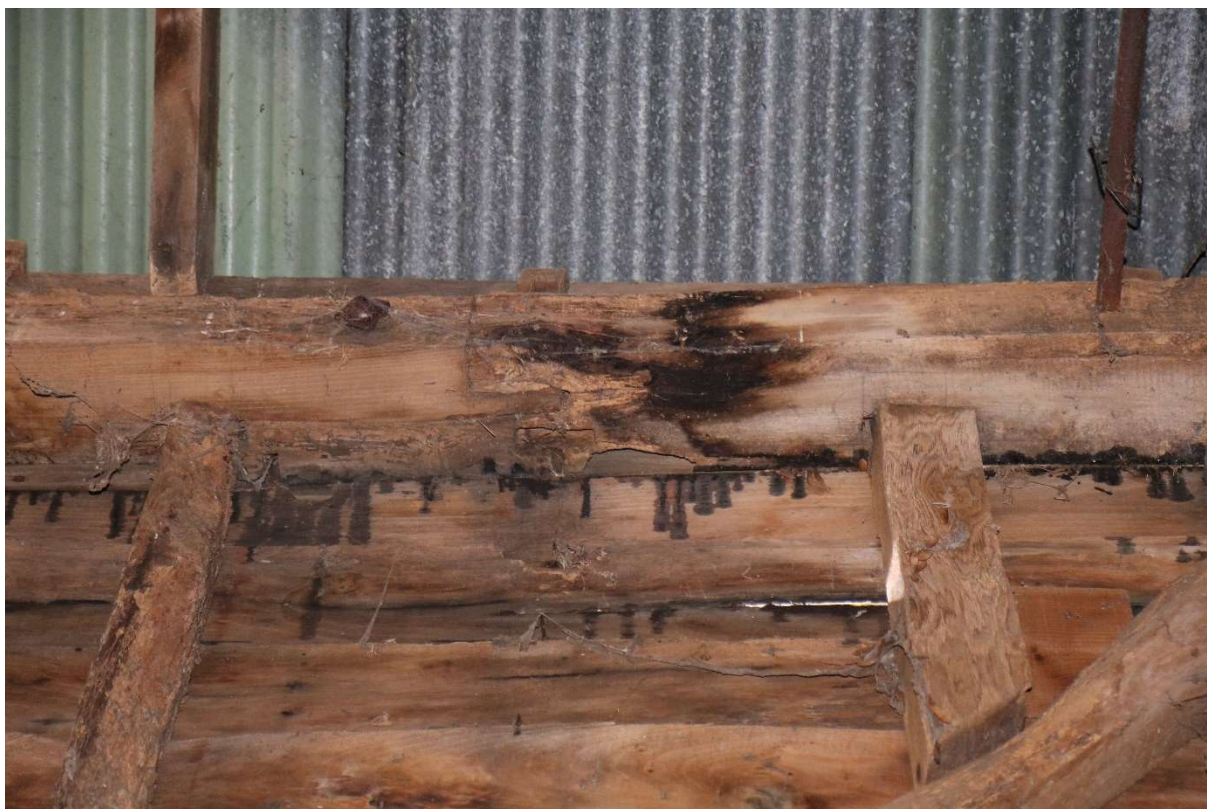
Photograph 19 Detail of scarf joint in wall-plate of north-western wall of bay 2 of threshing barn A. Photograph taken facing west north-west.
