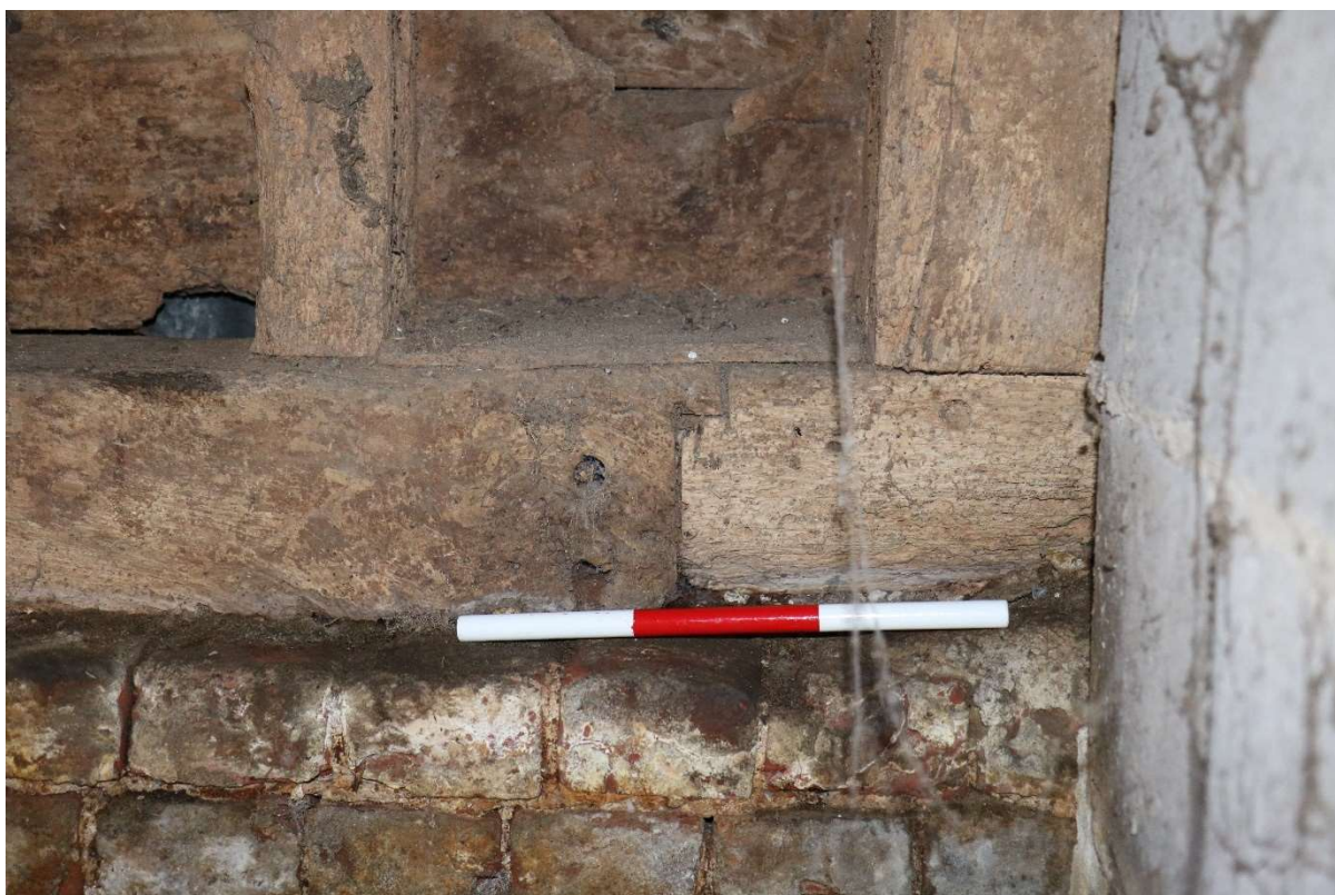
Photograph 20 Detail of scarf joint in sill-beam of south-eastern wall of bay 2 of threshing barn A. Photograph taken facing east south-east.
