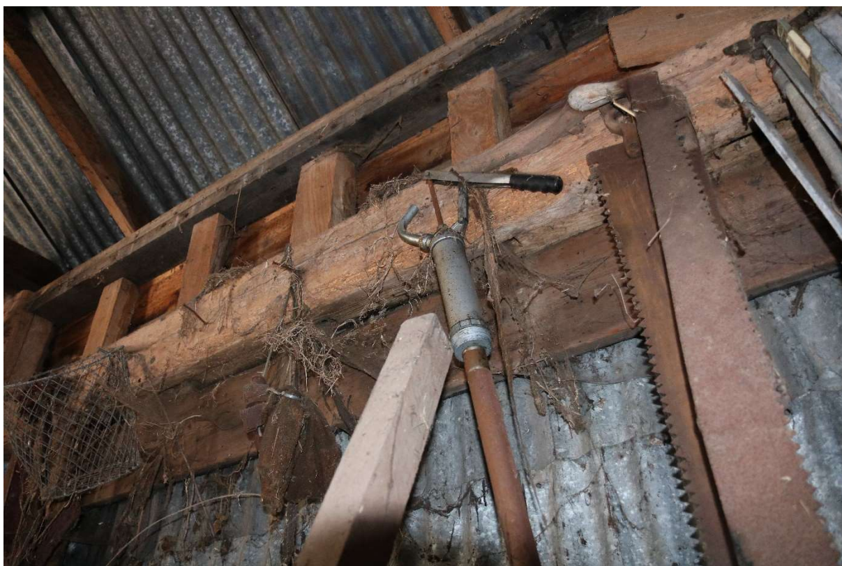
Photograph 38 Detail of empty mortices indicating inserted doorway in north-eastern wall of bay 3 of threshing barn B. Photograph taken facing north.
