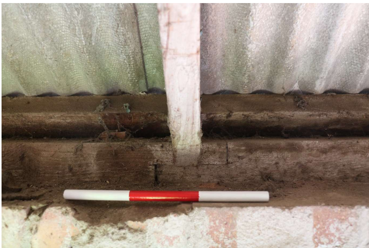
Photograph 50 Detail of scarf joint in wall-plate in south-western wall of brick shed. Photograph taken facing south-west.
