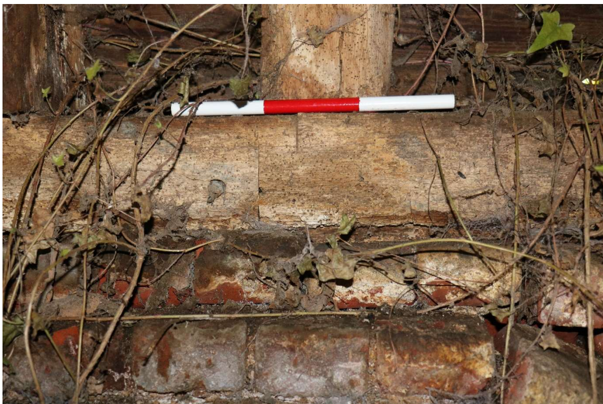
Photograph 27 Detail of scarf joint in sill-beam on north-western wall of bay 5 of threshing barn A. Photograph taken facing west north-west.
