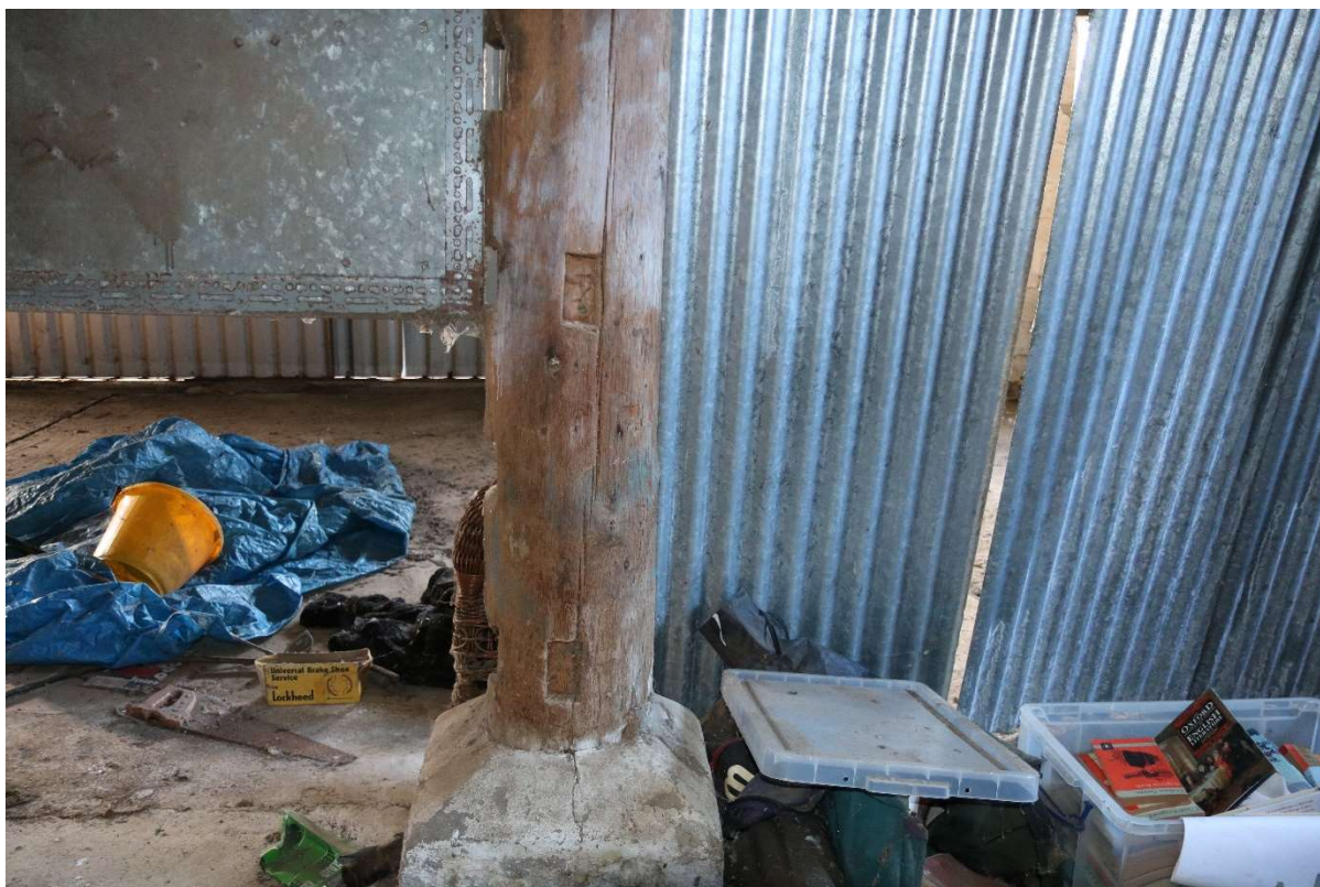
Photograph 46 Detail of reused centre-post of linking shed. Photograph taken facing west.
