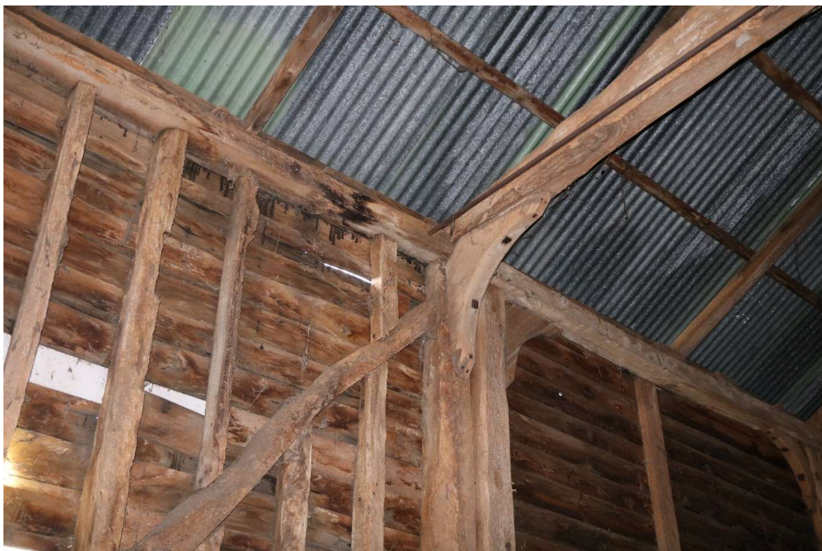
Photograph 15 Detail of knee brace and iron tie rod in north-western wall of bay 2 of threshing barn A. Photograph taken facing north-west.
