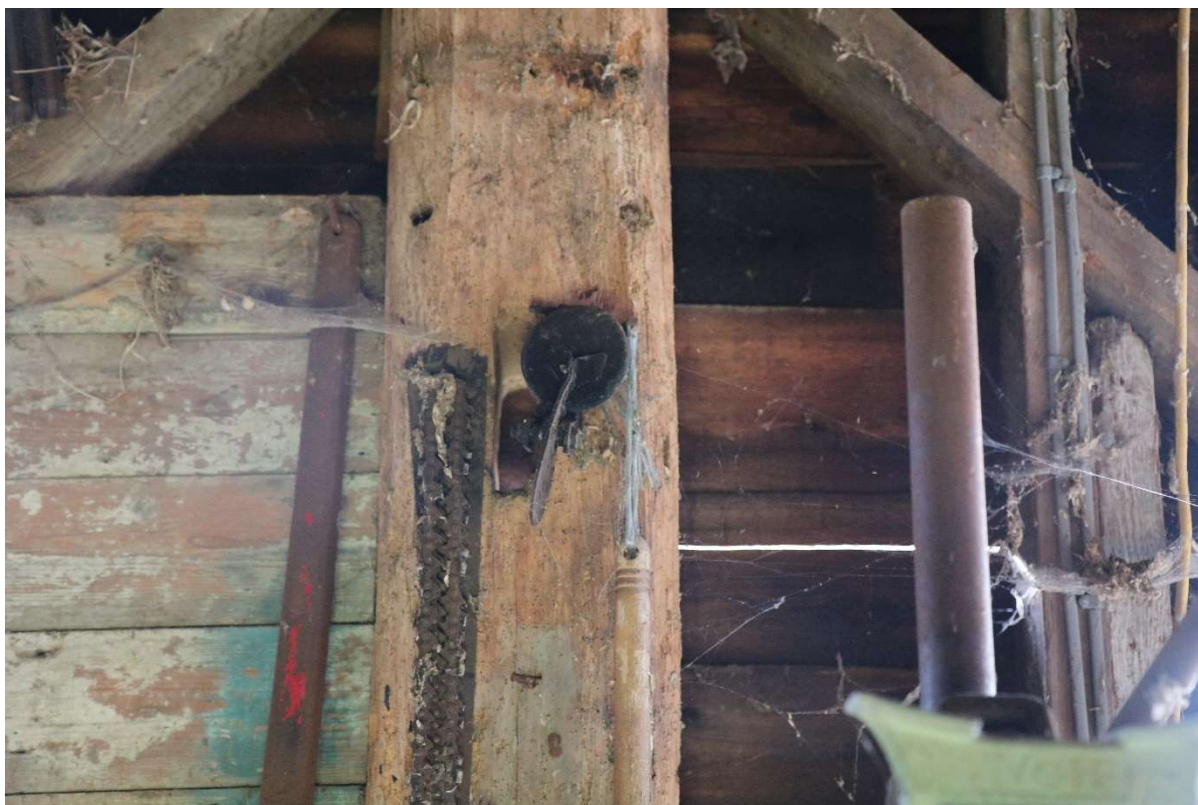
Photograph 34 Detail of reused intermediate post in south-western wall of bay 1 of threshing barn B. Photograph taken facing south-west.
