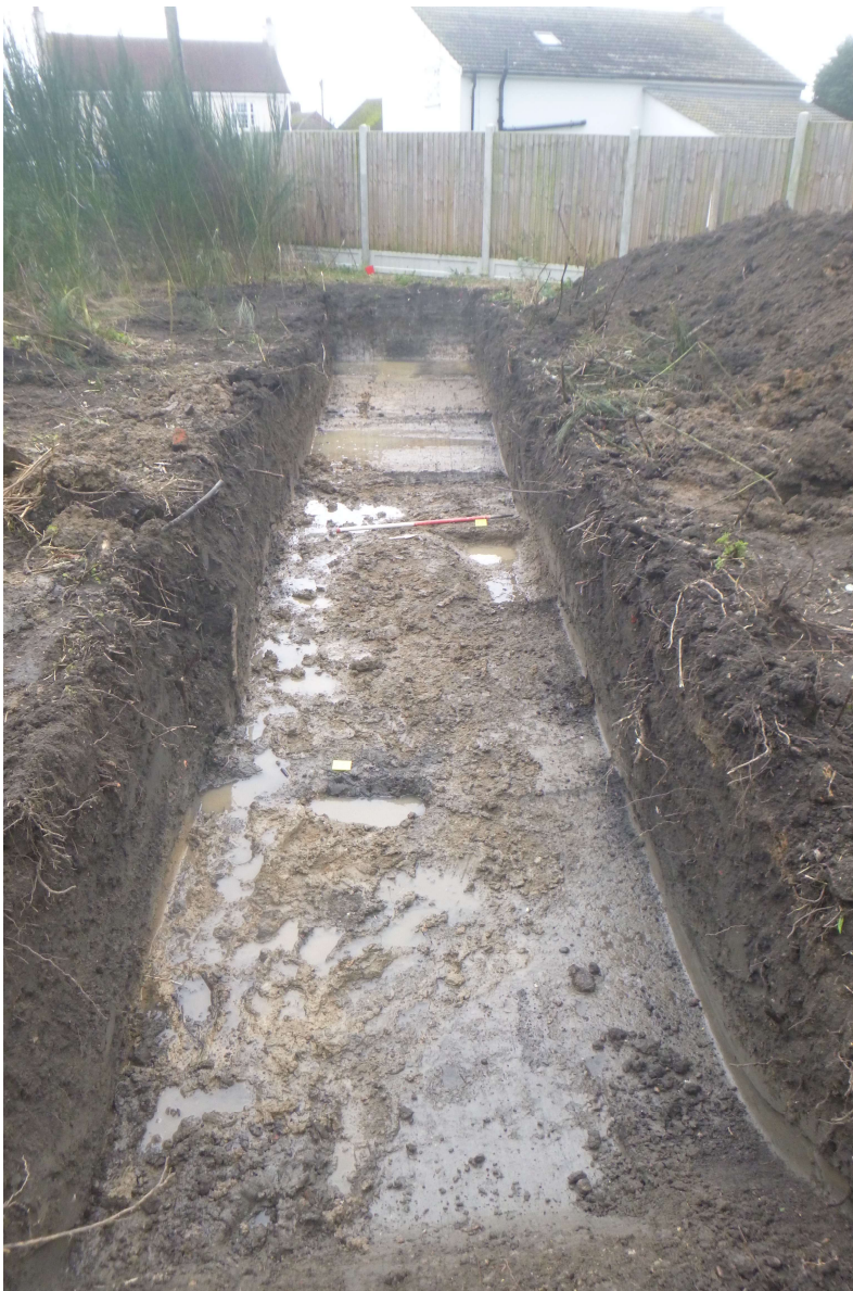
Photograph 1 The trench, looking south-east.
