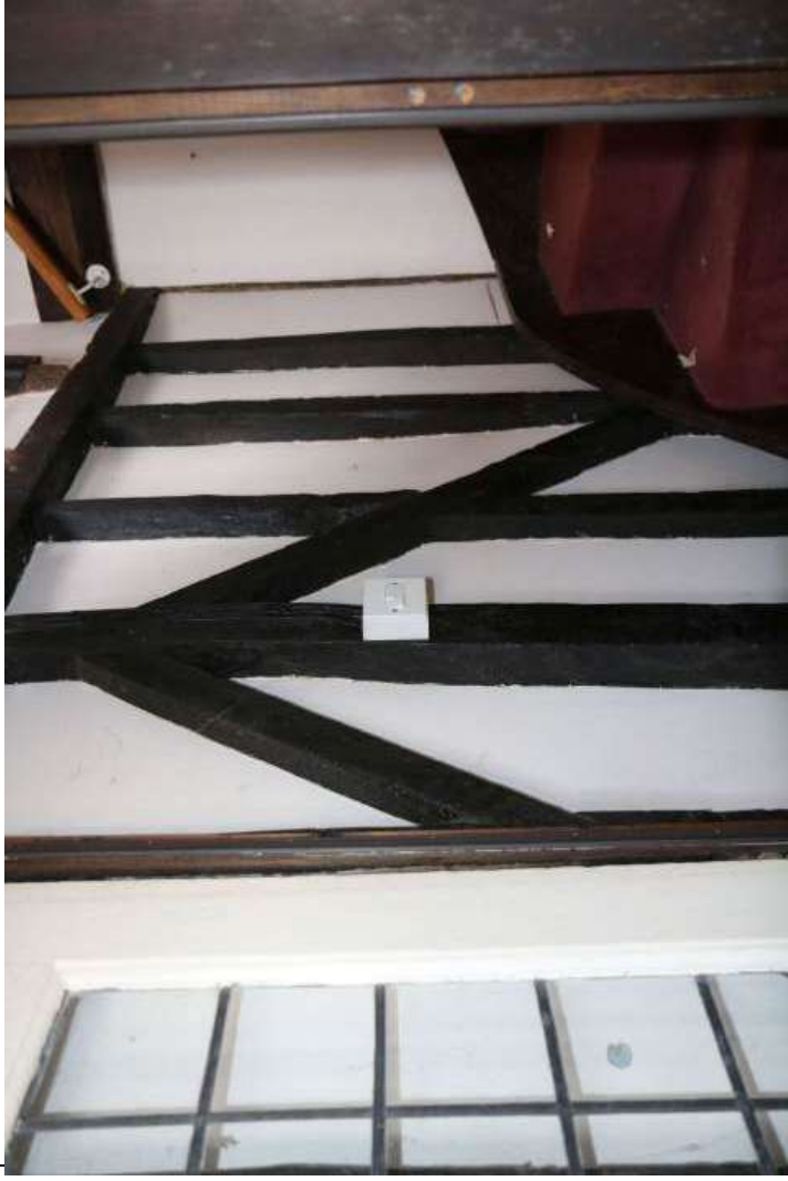
EEEX61395_PhotoGraph_0086 Detail of timber-framing in eastern wall of lounge stairs. Photograph taken facing south-east.
