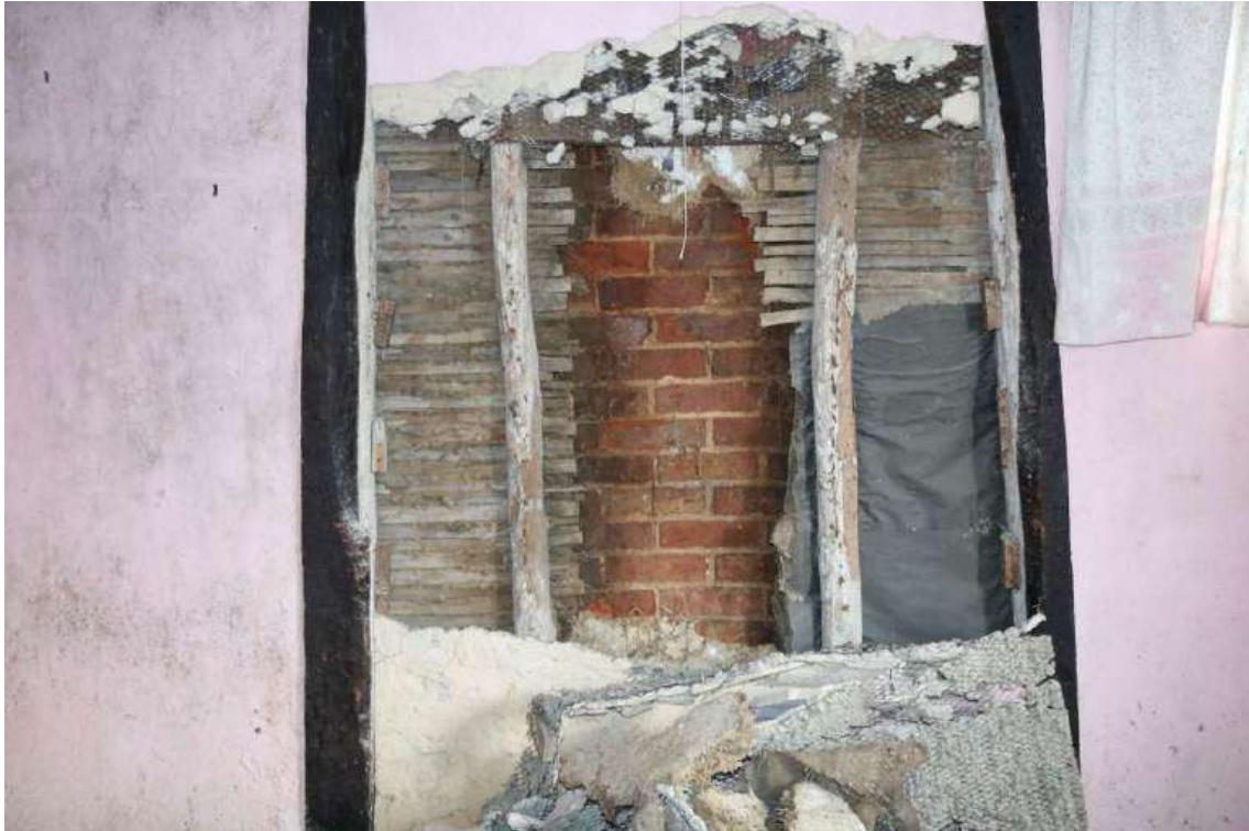
Photograph 32 Detail of plaster removal in western wall of bedroom 4, exposing brickwork of chimney. Photograph taken facing west.
