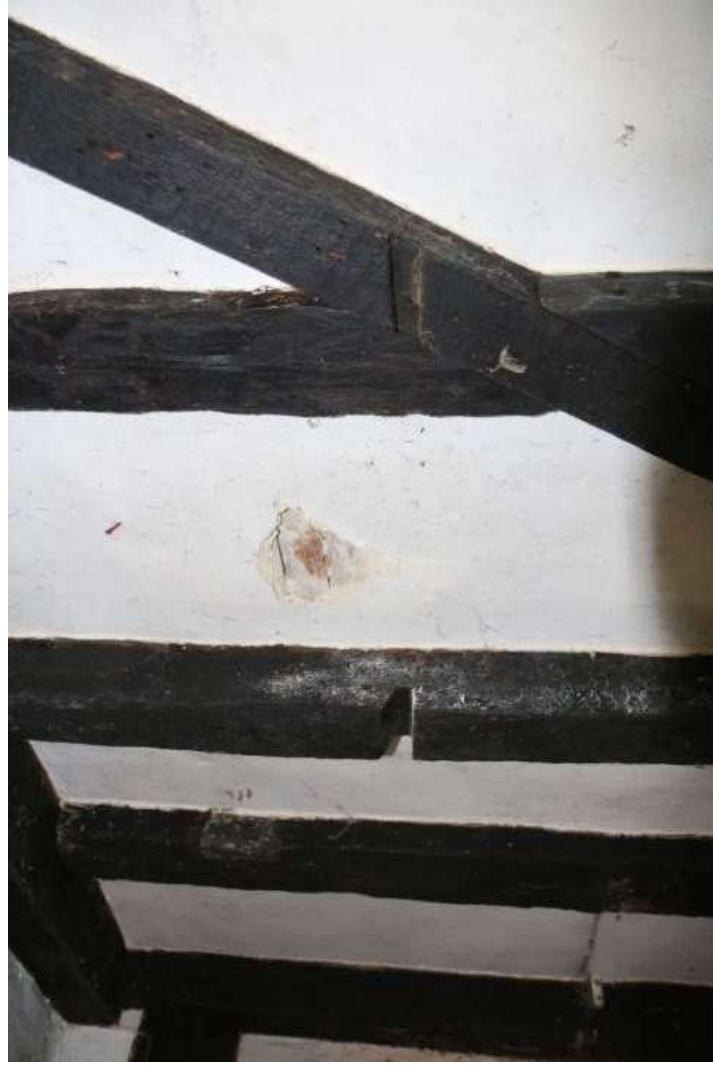
EEEX61395_Photo0076 Detail of possible evidence of reuse on stud and brace in northern wall of lounge. Photograph taken facing north-west.
