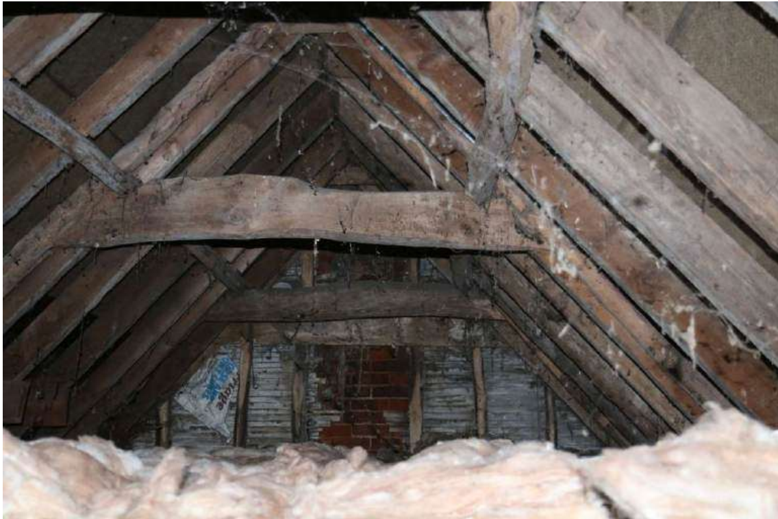
Photograph 11 Detail of original range roof construction. Photograph taken facing west.
