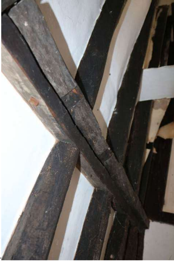
EEX61395_PhotoGraph_0082 Evidence of reused timber stair trimmer in ceiling of lounge. Photograph taken facing south-west.
