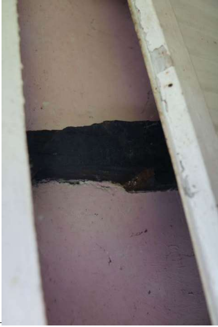
EEEX61395_PhotoGraph_0134 Detail of possibly reused timber in northern wall of bedroom 4, Photograph taken facing north north-east.
