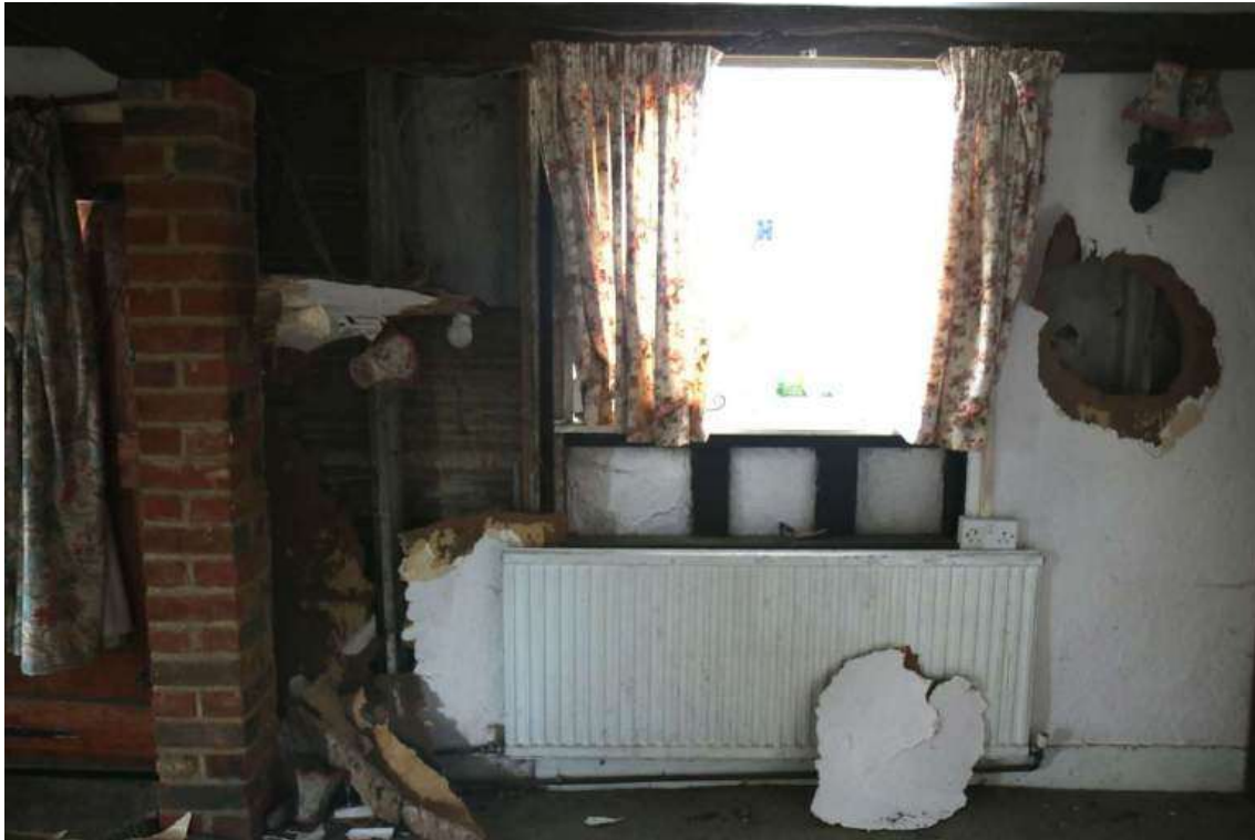
Photograph 21 Detail of replacement timber-framing in northern wall of lounge. Photograph taken facing north.
