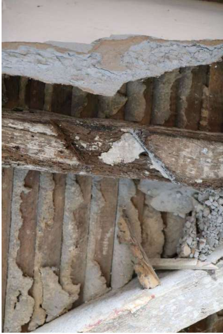
EEEX61395_Photograph_0039 Evidence of resuse on stud in northern wall of dining room. Photograph taken facing north.
