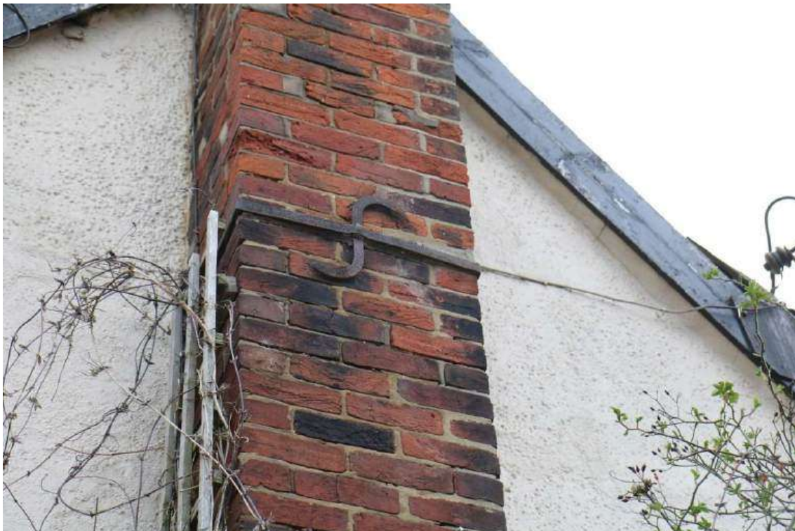
Photograph 6 Detail of iron strap and anchor plate on chimney breast on western elevation. Photograph taken facing south-east.
