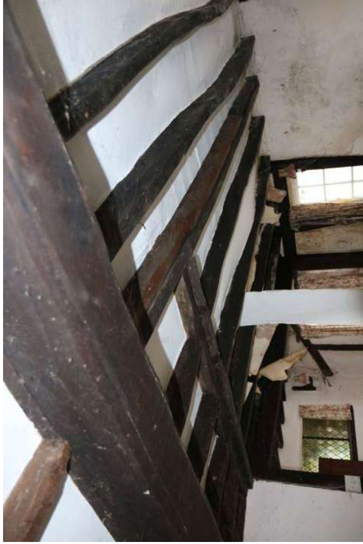
EEEX61395_Photograph_0079 Detail of floor joists, stair trimmer and sheathed binding beam in ceiling of lounge. Photograph taken facing south-west.
