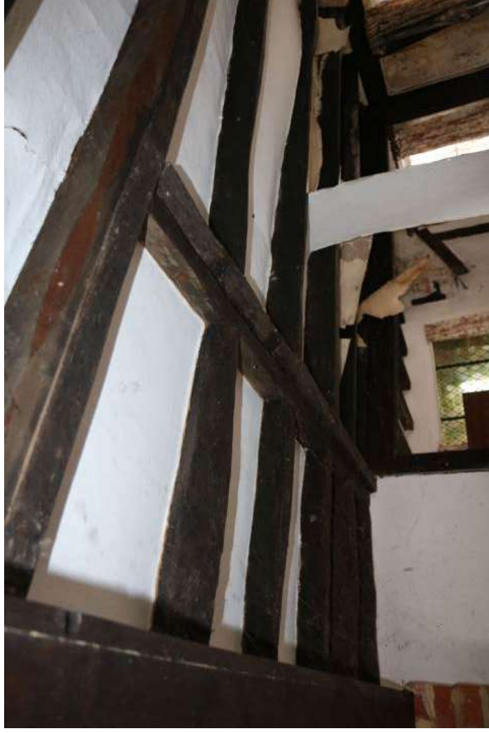
EEEX61395_Photograph_0080 Detail of floor joists and stair trimmer in ceiling of lounge. Photograph taken facing south-west.
