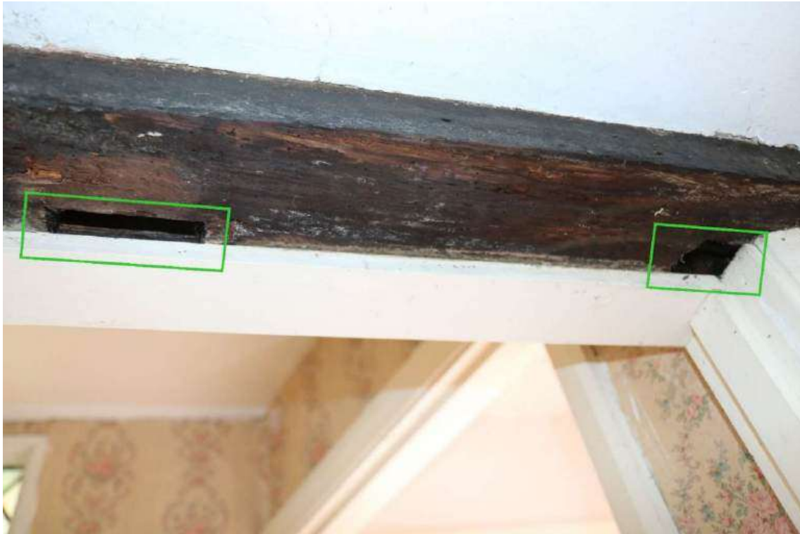
Photograph 35 Detail of empty mortices, highlighted in green, in southern wall-plate of bedroom 4. Photograph taken facing south-west.
