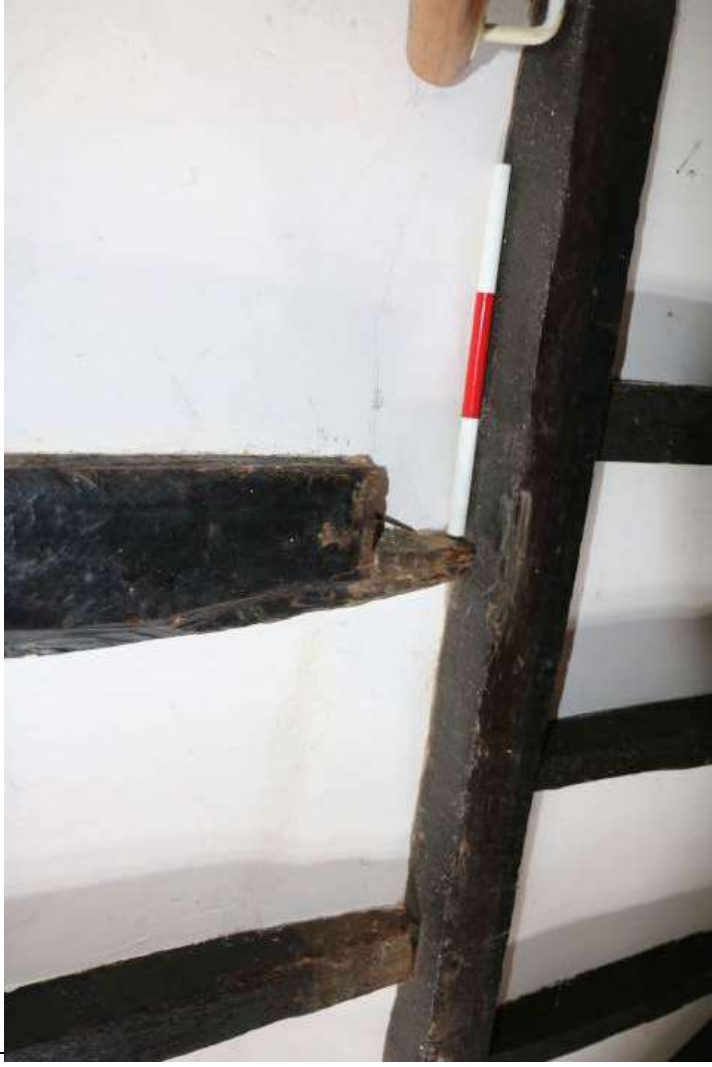
EEEX61395_PhotoGraph_0102 Detail of ?damaged timber in eastern wall of hall 1. Photograph taken facing east north-east.
