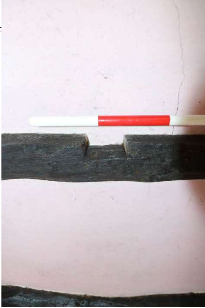
EEEX61395_PhotoGraph_0133 Detail of reused stud in northern wall of bedroom 4, Photograph taken facing north.
