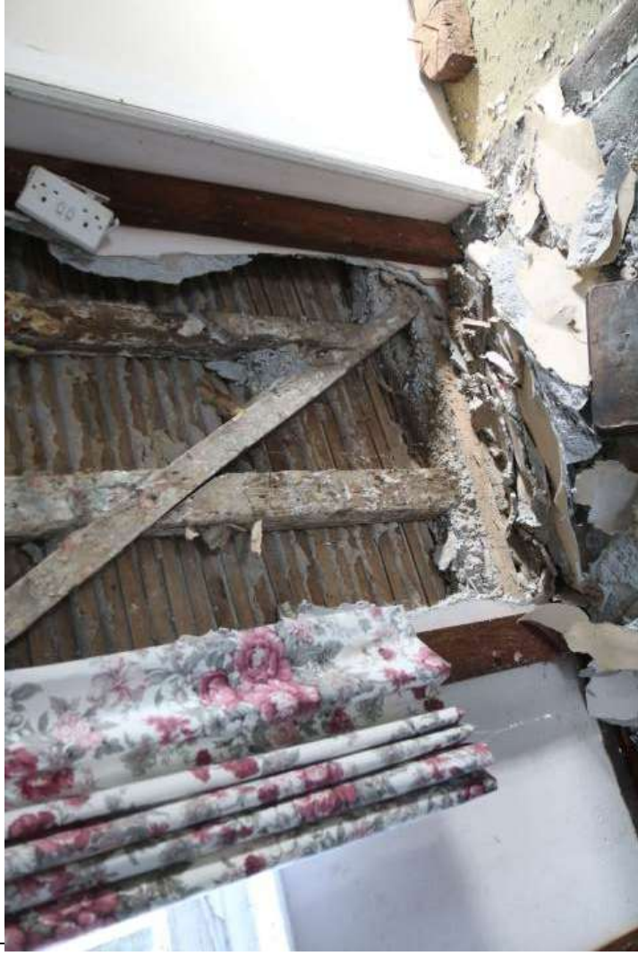
EEEX61395_Photograph_0038 Detail of sill-beam in northern wall of dining room. Photograph taken facing north north-east.
