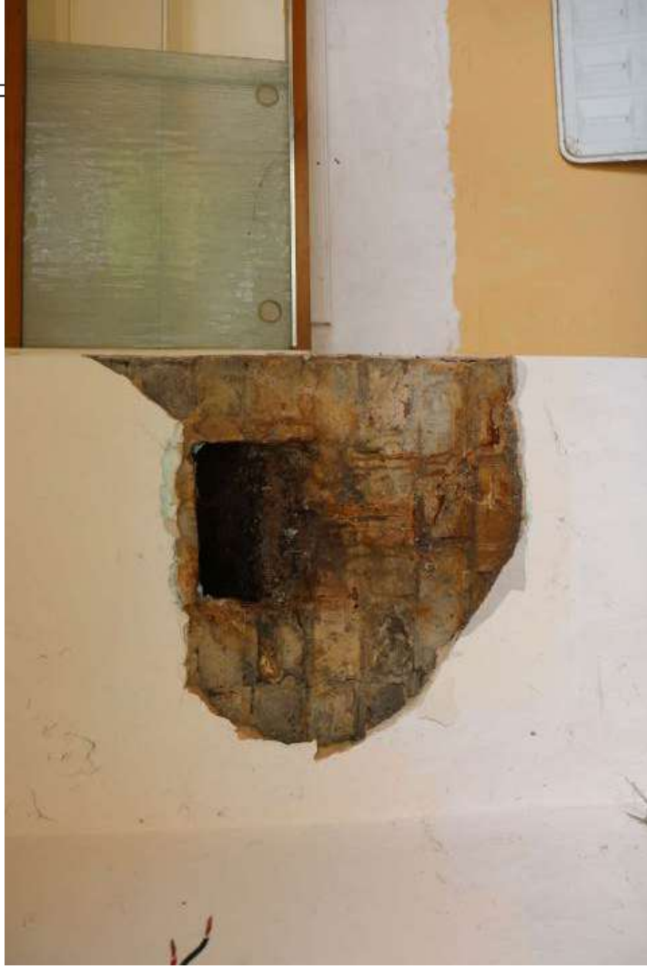
EEX61395_PhotoGraph_0057 Detail of exposed brick chimney in northern wall of utility room. Photograph taken facing north.
