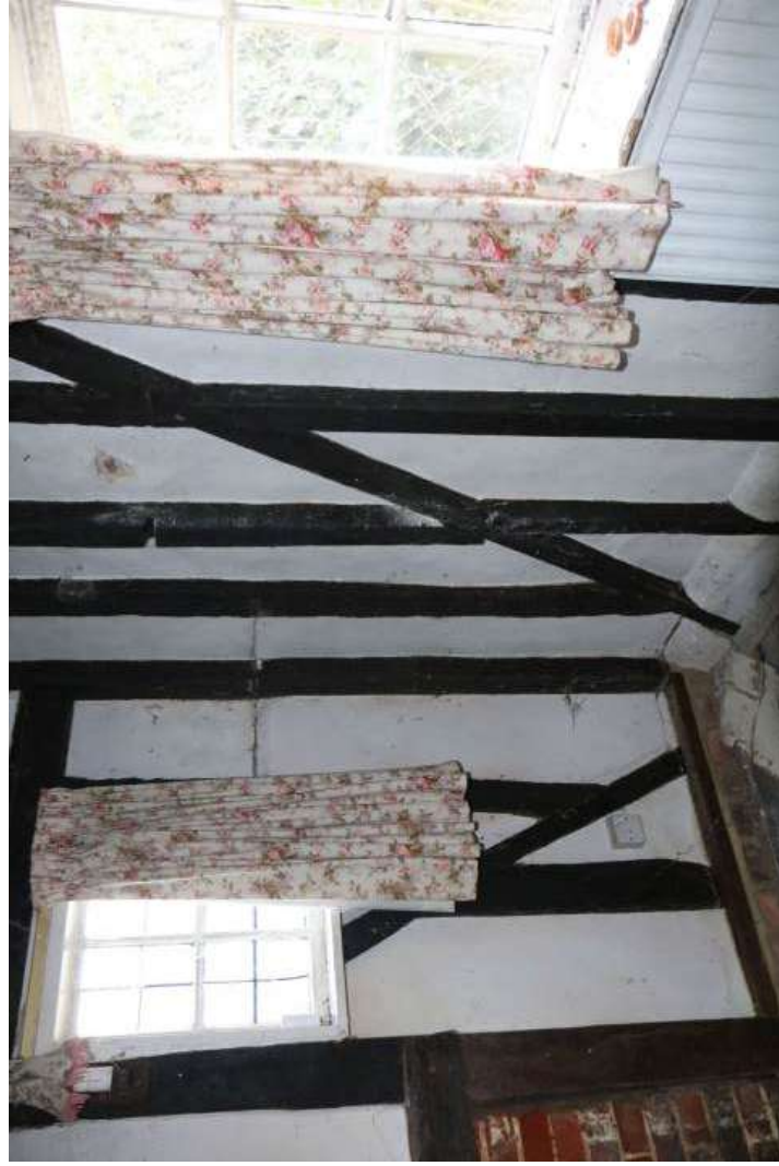
EEEX61395_Photo0075 Detail of timber-framing in northern and western walls of lounge. Photograph taken facing north-west.
