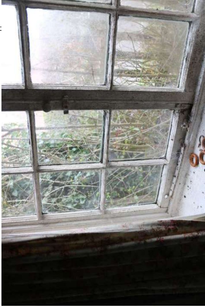
EEEX61395_Photograph_0065 Detail of window catch and stay in northern wall of lounge. Photograph taken facing north-west.
