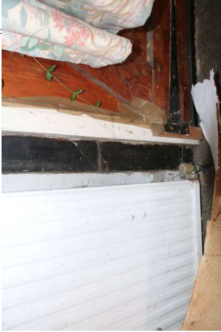
EEX61395_PhotoGraph_0081 Possible evidence of reuse in doorpost in northern wall of lounge. Photograph taken facing north.
