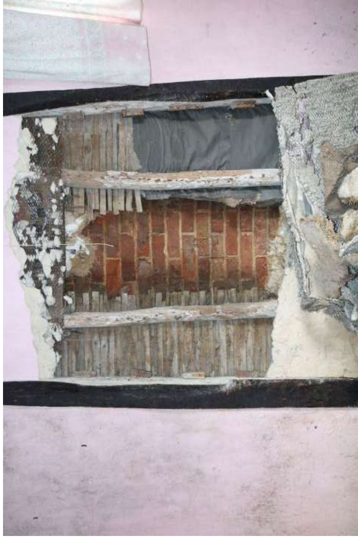
EEEX61395_Photograph_0143 Detail of plaster removal in western wall of bedroom 4, exposing brickwork of chimney. Photograph taken facing west.
