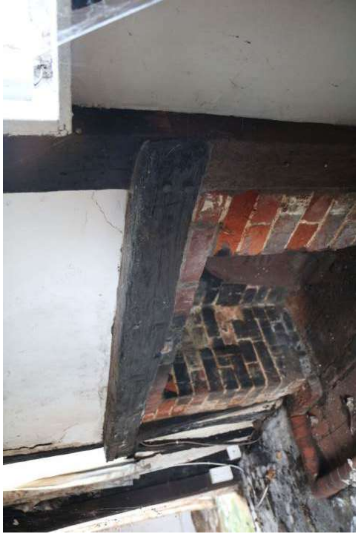
EEEX61395_PhotoGraph_0072 Detail of timber lintel above fireplace in western wall of lounge. Photograph taken facing south-west.
