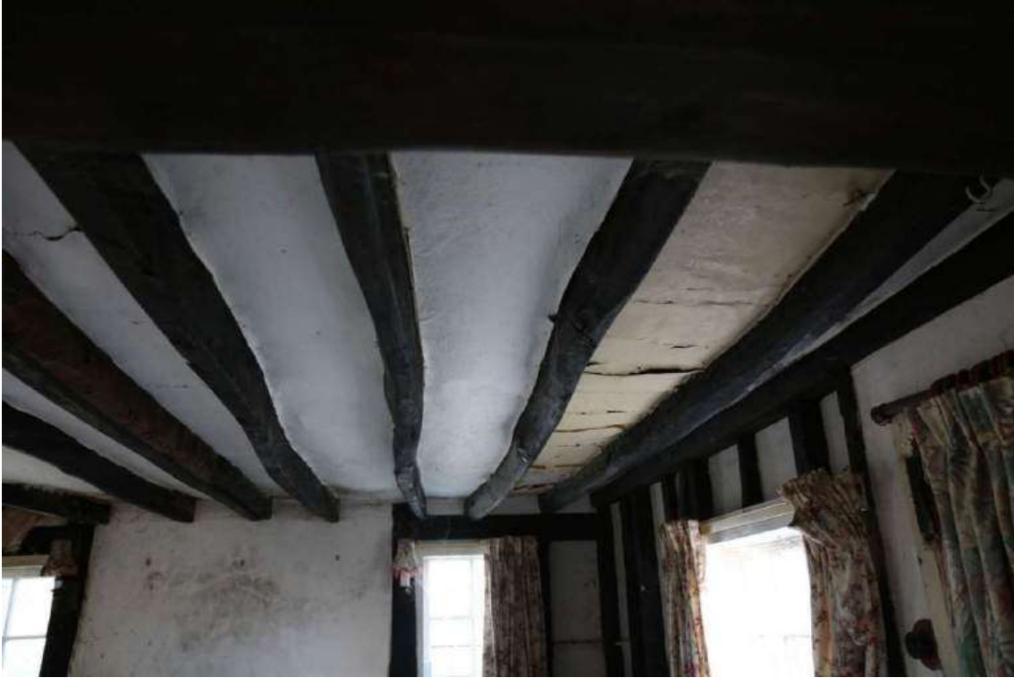
Photograph 23 Detail of floor joists in ceiling of lounge. Photograph taken facing west.
