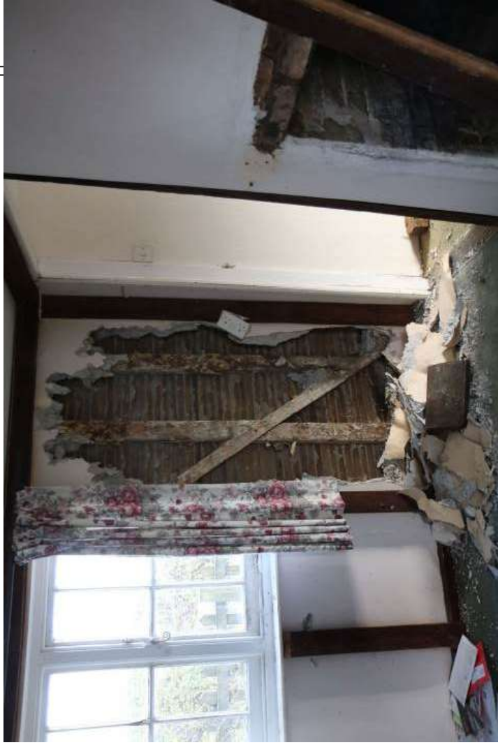
EEEX61395_Photograph_0037 Detail of exposed timber-framing in northern wall of dining room. Photograph taken facing north north-east.
