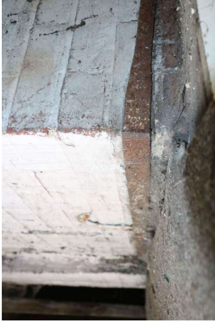
EEEX61395_PhotoGraph_0139 Detail of iron strap and plate on brick chimney breast in attic space above bedroom 1. Photograph taken facing south-west.
