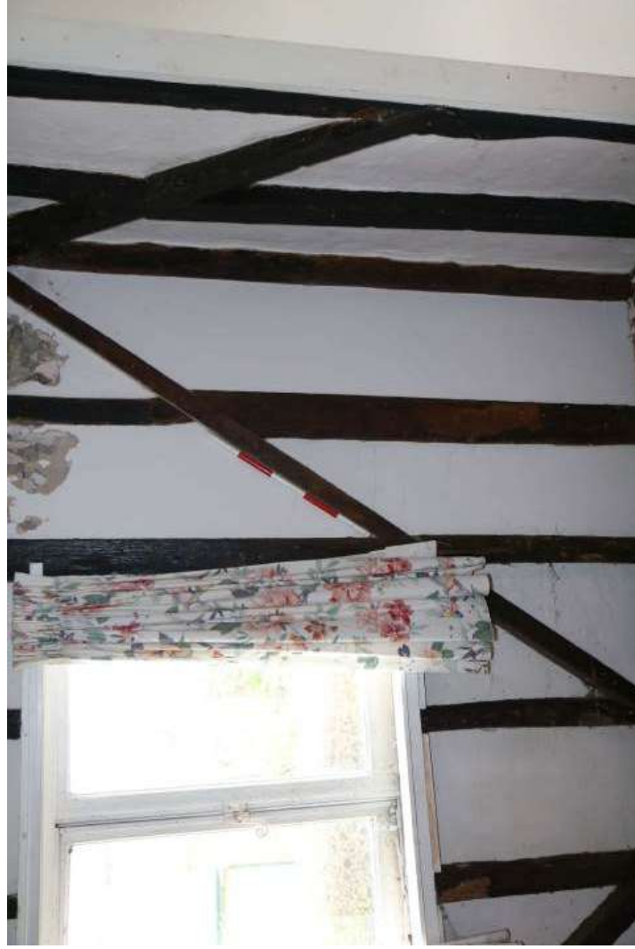
EEEX61395_Photograph_0099 Detail of timber-framing in northern wall of hall 1. Photograph taken facing north.
