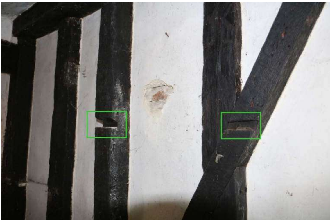
Photograph 20 Detail of possible evidence of reuse on stud and brace in northern wall of lounge. Photograph taken facing north-west.
