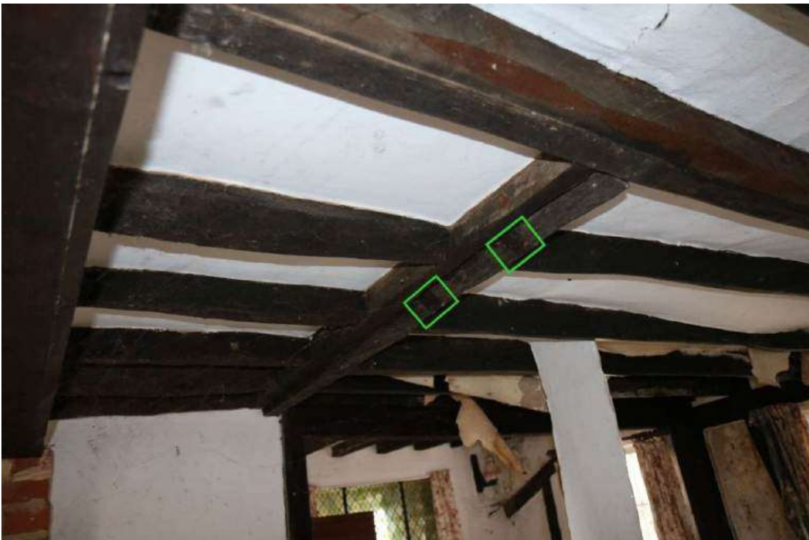
Photograph 24 Detail of floor joists and stair trimmer in ceiling of lounge. Evidence of reuse on the stair trimmer highlighted in green. Photograph taken facing south-west.
