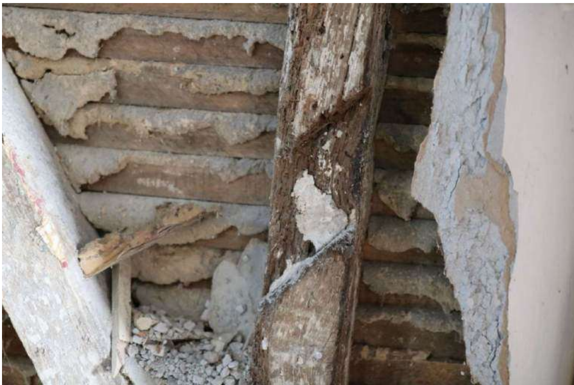
Photograph 17 Evidence of reuse on stud in northern wall of dining room. Photograph taken facing north.
