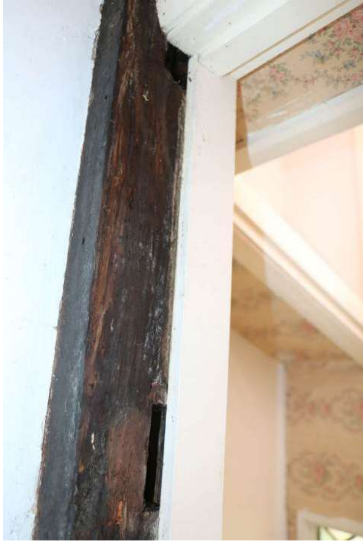
EEEX61395_PhotoGraph_0136 Detail of empty mortices in southern wall-plate of bedroom 4, Photograph taken facing south-west.
