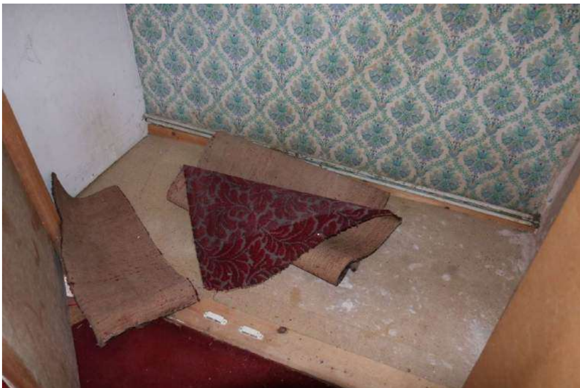
Photograph 34 Detail of modern sheet timber floor in southern cupboard in bedroom 4. Photograph taken facing north-east.
