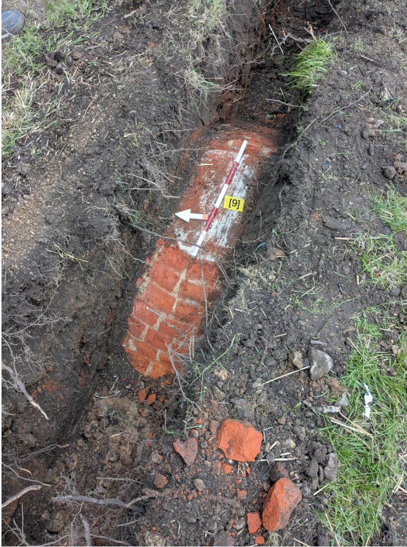
Photograph 2 Brick soakaway [9], view north-east.
