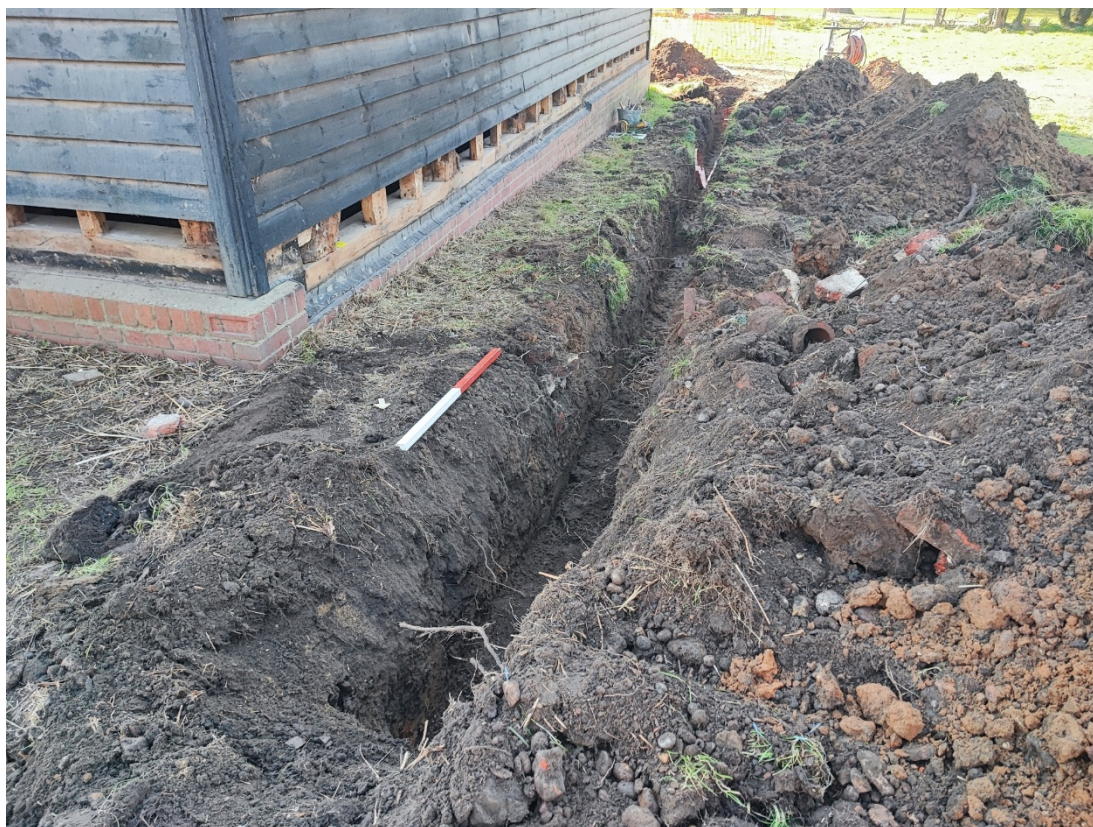
Photograph 4 Trench to the west of the barn, view south south-west.
