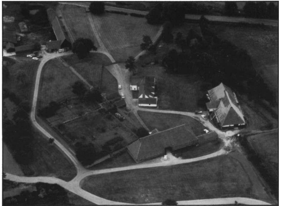
Cressing Temple from the air showing the Barley Barn (centre right) under repair and excavations in progress at the far end of the walled garden (centre left).
