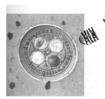
Iron was, and still is, often used for sturdy covers set into pavements or roads. This is a coalhole cover in the pavement outside a house. Sacks of coal were tipped through here into the cellar of the house.
