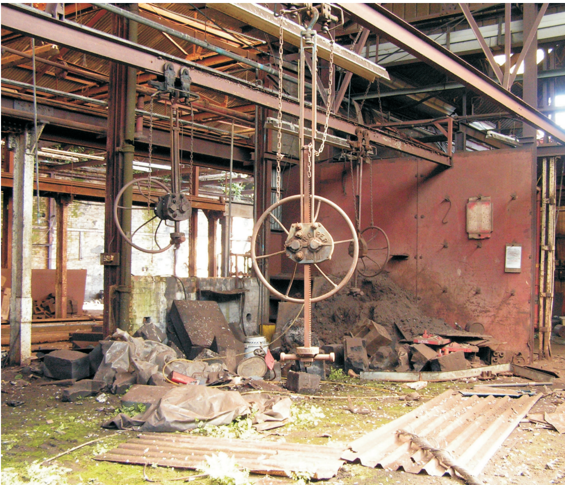
Ladle hoists attached to the overhead metal-handling monorail.
