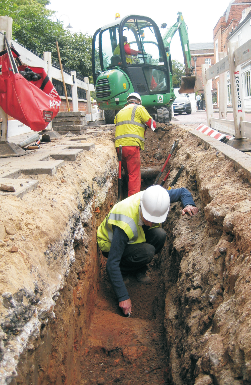
Don Shimmin uncovers Boudica's handiwork in Queen Street.
