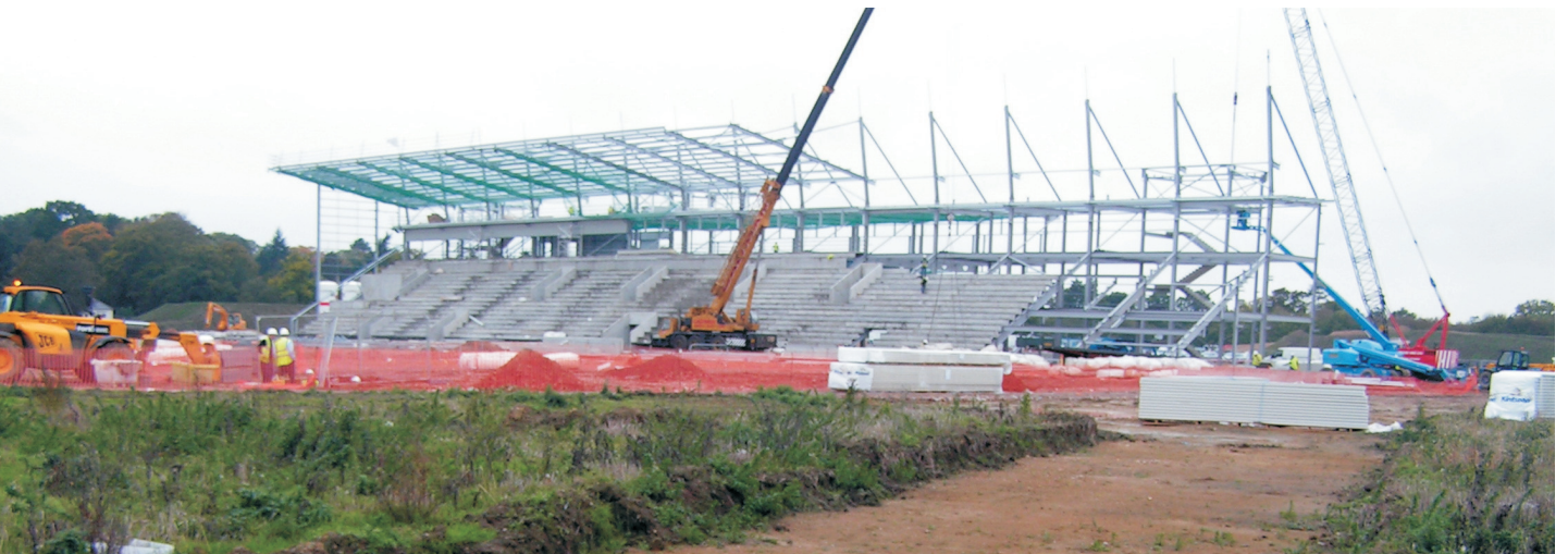
Colchester United's stadium under construction.
