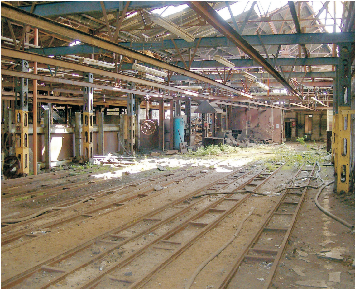
The casting floor with the embedded rails to move moulds along beneath the monorail.
